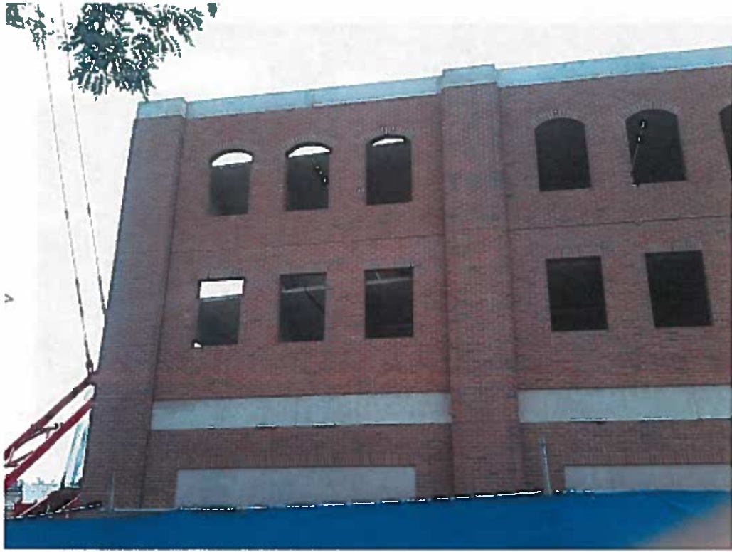
"Flanagan Panels" Along 4 th and Cotanche Streets.
