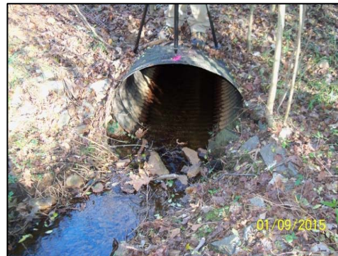
Picture 4-1: King George Road Culvert – Upstream Face
