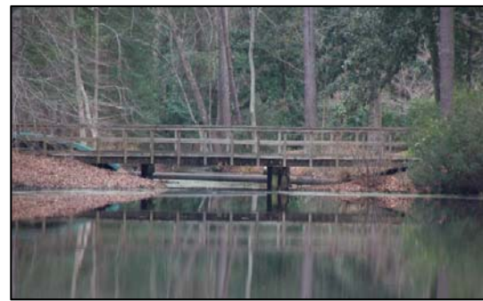
Picture 3-4: Holly Hills Road Bridge – Downstream Face
