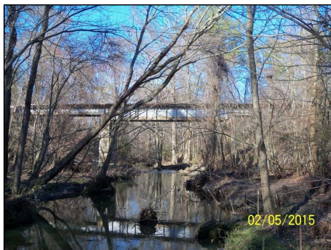
Picture 4-2: Railroad Trestle - Upstream Face
