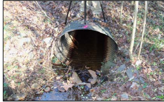
Picture 3-6: King George Road Culvert – Downstream Face
