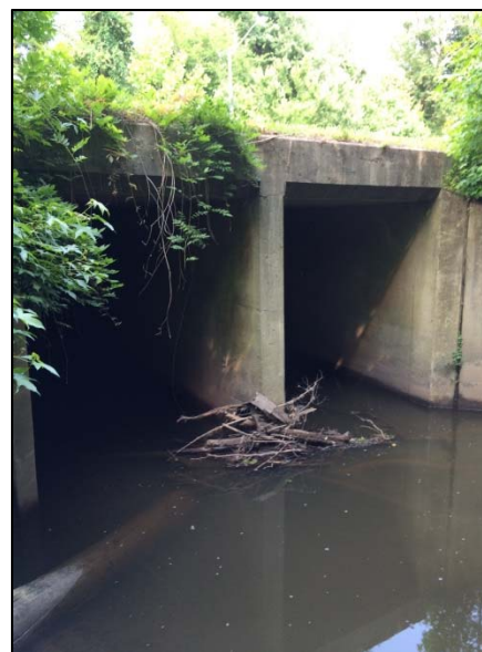
Picture 4-3: E 10th Street - Upstream Face
