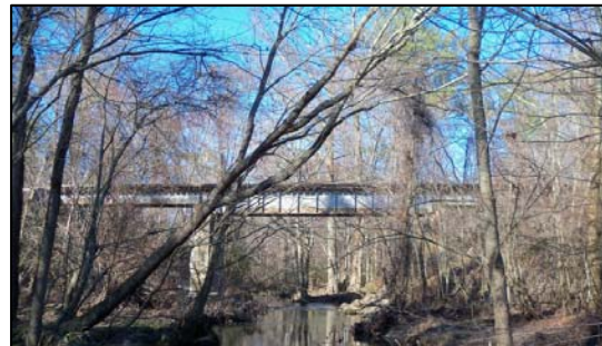
Picture 3-2: Railroad Crossing Bridge – Downstream Face
