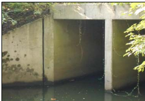
Picture 3-3: East 10 th Street Culvert – Downstream Face
