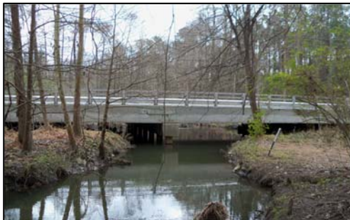
Picture 3-1: Portertown Road Bridge – Downstream Face
