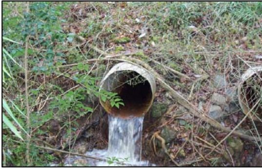
Picture 3-5: Cardinal Drive Culvert – Downstream Face
