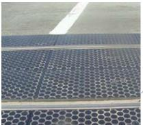
Installing a rubber surface rather than asphalt around railroad flangeways reduces changes in level and other maintenance problems.
