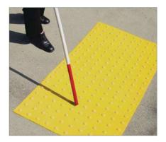
The use of texture and bright color at curb ramps helps the visually impaired to cross safely.
