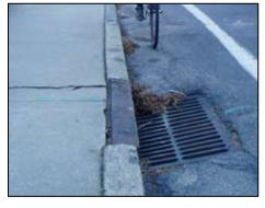
Dangerous Drainage Grate Condition; this example is dangerous due to the surrounding paring condition (when the road was resurfaced the drainage grate remained at the same height).
