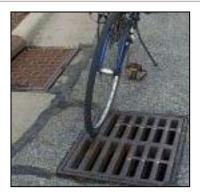
Dangerous Drainage Grate Condition; this example is dangerous due to the grate running parallel to the roadway, creating a trap for bicycle tires.
