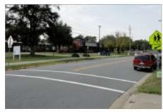
South Greenville Elementary crossing - lacks curb ramps, in-roadway signage, high-visibility marked crosswalk, and bulbouts
