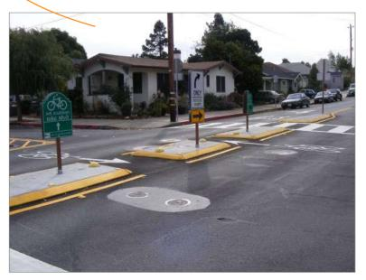
Bikeway planners and engineers may pick and choose the appropriate mix of design elements needed for bicycle boulevard development along a particular corridor. Mix and match design elements to:
