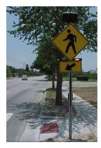
Left: RRFB with two forward-facing LED flashers and a side-mounted LED flasher.
