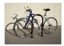
A single inverted " U" rack can accommodate two bicycles.
