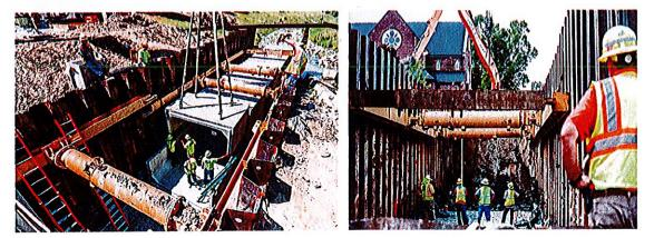
Once the 3<sup>rd</sup> Street RCBC was placed, Trader Construction began removing the existing arch culvert between 3<sup>rd</sup> Street and 4<sup>th</sup> Street making the new RCBC live and operational.
