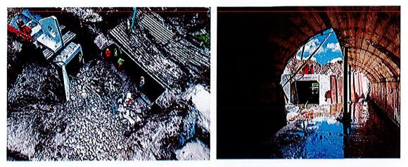
The second of six (6) SCM's was installed just north of 3<sup>rd</sup> Street. This is a small Regenerative Stormwater Conveyance (RSC) that drains the northern ECU parking lot to Town Creek. Following the completion of the small RSC, 3<sup>rd</sup> Street opened at the beginning of November.
