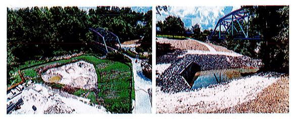
Shortly thereafter, the contractor began excavating and placing the 10'x8' reinforced concrete box culvert (RCBC) under 3<sup>rd</sup> Street. The floor of the new culvert is approximately 19 feet deep as seen in the pictures below.
