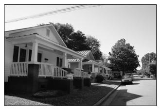
Photo 14: 601-605 Contentnea Street – typical rehabilitated houses with vinyl windows and new metal roofs
