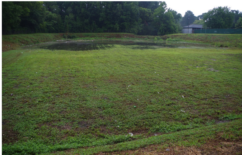
Photograph 5-12. Proposed Location for Moyewood Wet Pond Repair
