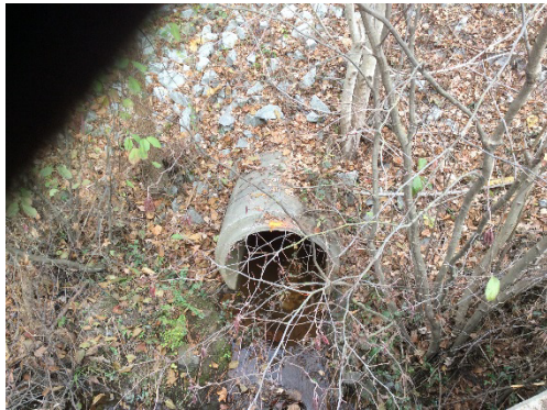
Photograph 3-9 Schoolhouse Branch: Pipe West of Arlington Boulevard – Downstream
