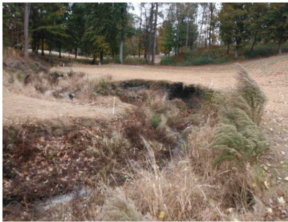
Photograph 5-3: Bank Erosion on Right Bank Facing Downstream
