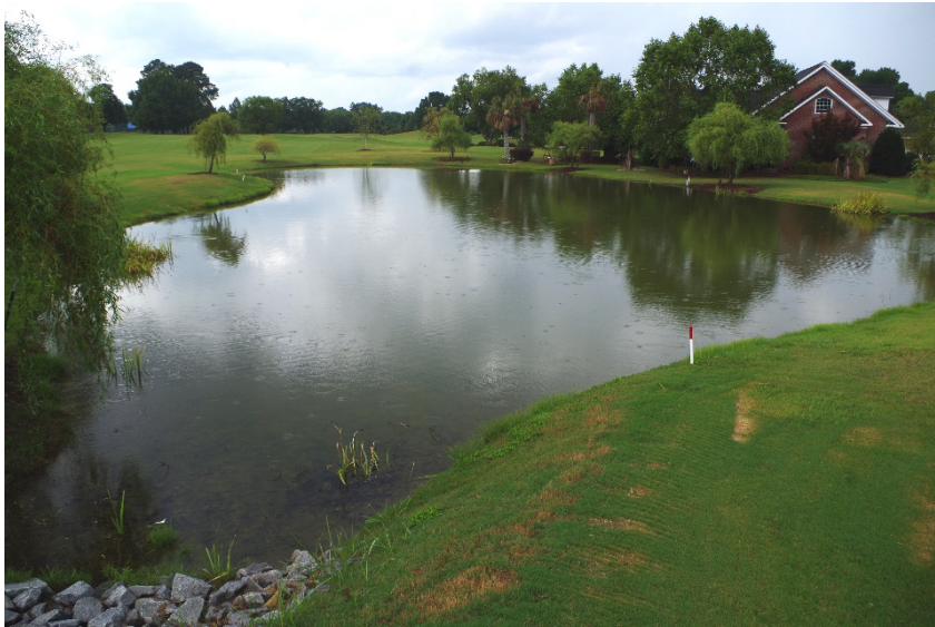
Photograph 5-10. Proposed Location for Ironwood Golf Course Wet Pond Retrofit– Downstream Pond
