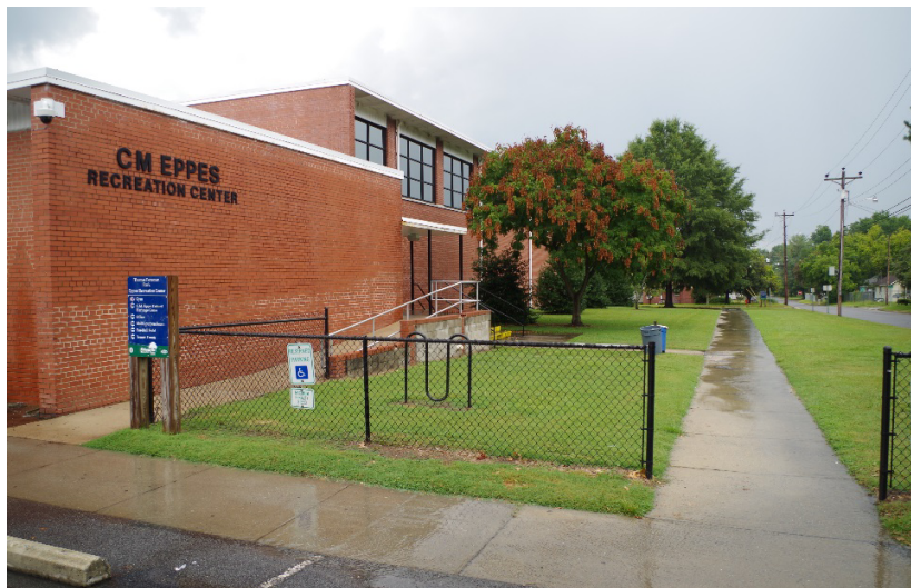
Photograph 5-13: Proposed Location for Thomas Foreman Park Bioretention
