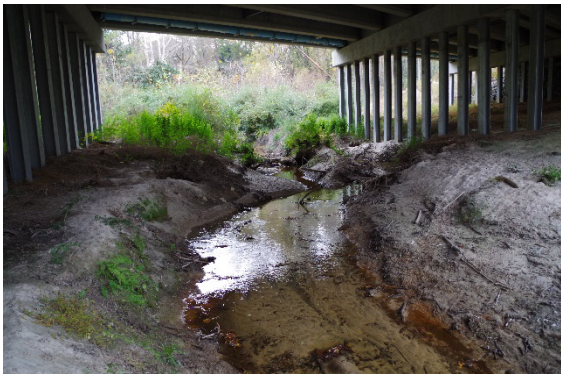
Photograph 3-1 Harris Mill Run: NC 43 Bridge – Upstream
