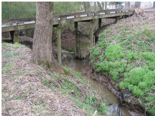
Photograph 3-15 Sams Branch: Ironwood Golf Cart Bridge 4
