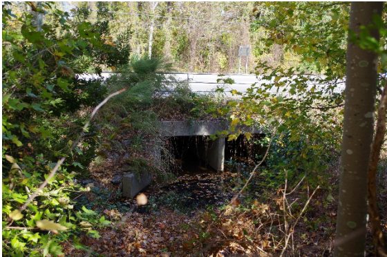
Photograph 3-3 Schoolhouse Branch: W 5 th Street Culvert
