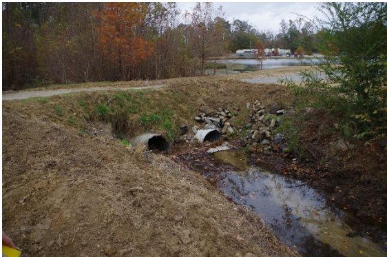
Photograph 3-18 Sams Branch: Maintenance Road Culvert Upstream
