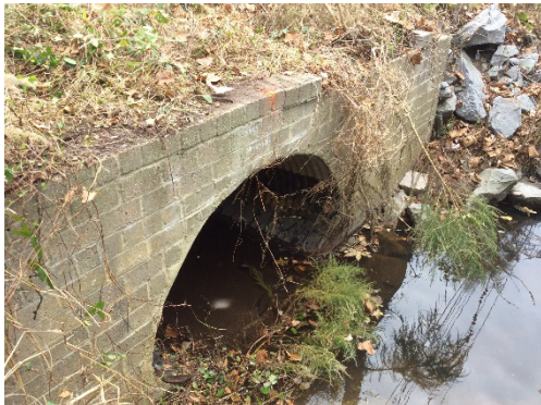
Photograph 3-5 Schoolhouse Branch: W 5 th Street CMP Culvert – Upstream
