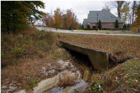
Photograph 3-17 Sams Branch: Golf View Drive Culvert Upstream
