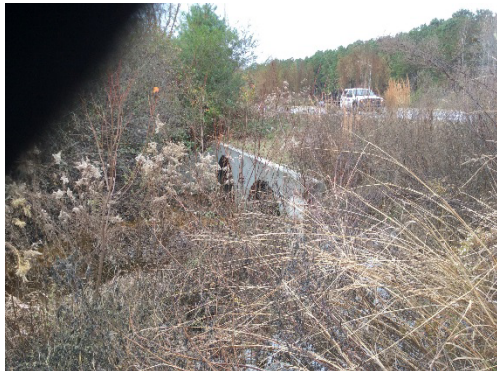
Photograph 3-7 Schoolhouse Branch: Arlington Boulevard Culvert – Downstream
