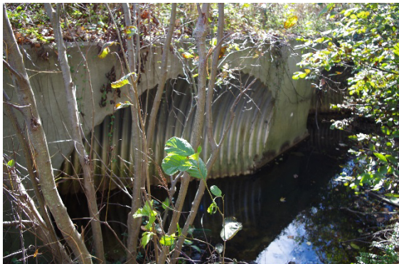
Photograph 3-4 Schoolhouse Branch: W Arlington Boulevard Culvert
