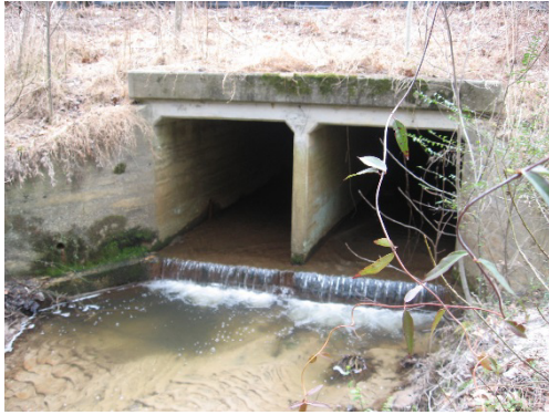
Photograph 3-19 Sains Branch: NC-43 Culvert Downstream
