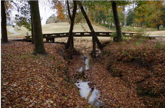
Photograph 3-12 Sams Branch 1: Ironwood Golf Cart Bridge 1
