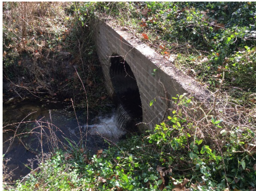
Photograph 3-6 Schoolhouse Branch: W 5 th Street Culvert – Downstream
