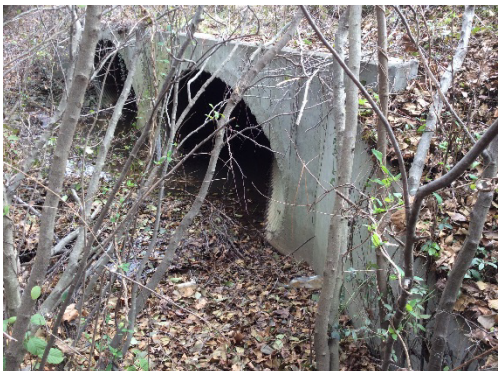
Photograph 3-8 Schoolhouse Branch: Arlington Boulevard Culvert – Upstream
