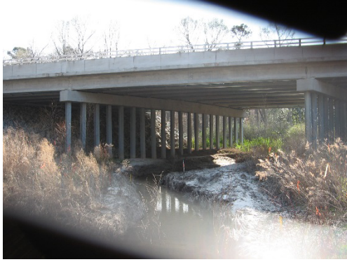
Photograph 3-2 Harris Mill Run: NC 43 Bridge – Downstream
