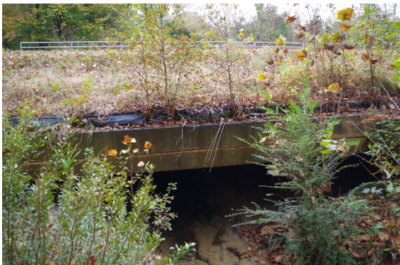
Photograph 3-16 Sams Branch 1: Golf View Drive Culvert – Downstream
