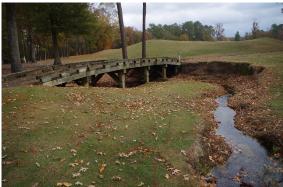
Photograph 3-14 Sams Branch: Ironwood Golf Cart Bridge 3
