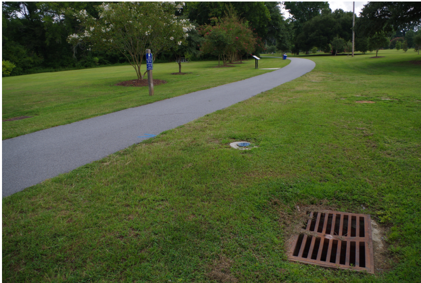
Photograph 5-17: Proposed Location for S Tar River Greenway Pipe Daylighting
