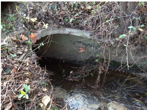
Photograph 3-10 Schoolhouse Branch: Pipe West of Arlington Boulevard – Upstream
