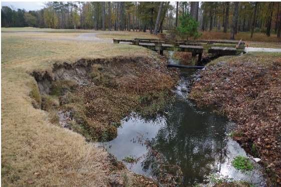
Photograph 3-13 Sams Branch 1: Ironwood Golf Cart Bridge 2
