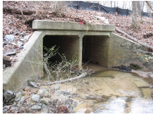
Photograph 3-20 Sains Branch: NC-43 Culvert Downstream
