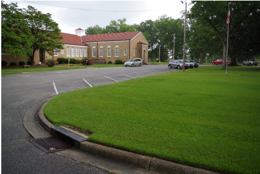
Photograph 5-15: Proposed Location for Third Street Community Center Bioretention Area
