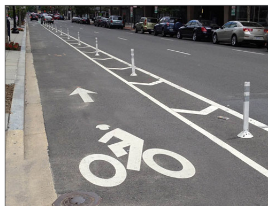
Separated Bikeway, Washington, D.C - Photo from FHWA
