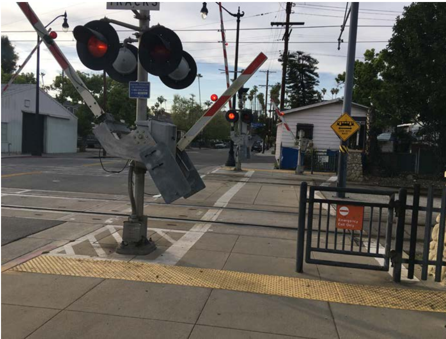
A pedestrian crossing in Los Angeles on the Metro Gold Line includes automatic pedestrian gates and emergency exit swing gates. Where geometrically feasible, they are attached to the same assembly as the roadway gates for cost savings.
