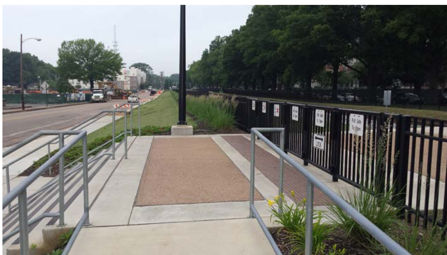
This pedestrian rail crossing at the University of Memphis uses pull gates to encourage pedestrians to look for trains before crossing the tracks. The exit gates to the left of the entrance gates prevent pedestrians from getting caught on the tracks.
