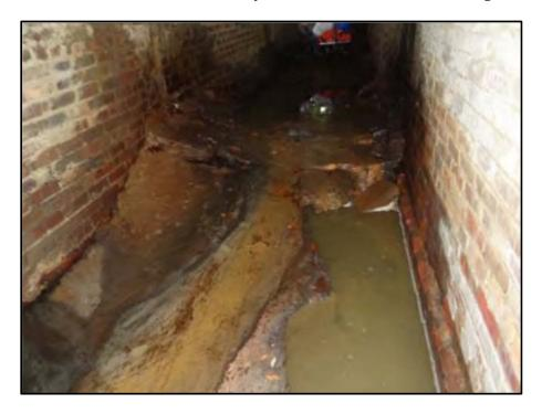
Photo 1: Floor Heaving and Cracking
