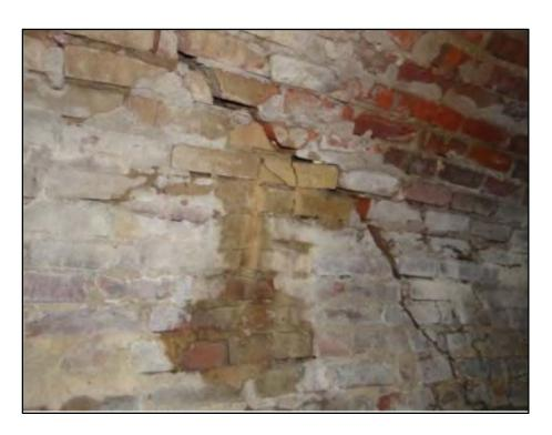
Photo 3: Brick Arch with Cracks
