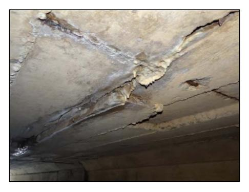
Photo 4: Concrete Box with Spalling and Exposed Steel
