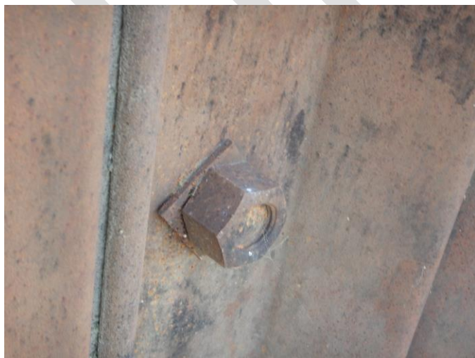
PHOTOGRAPH 2.5: TIE ROD NUT
