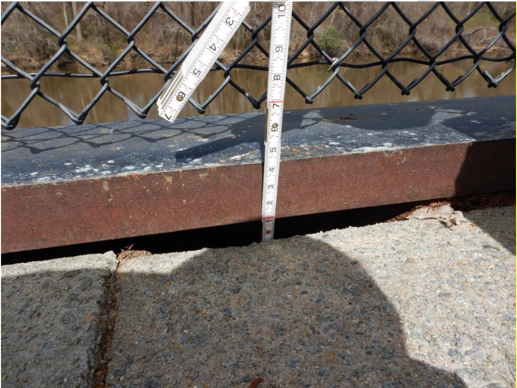
PHOTOGRAPH 2.2: SETTLEMENT OF SLAB AT EDGE OF BULKHEAD CAP (STATION 1+85)
