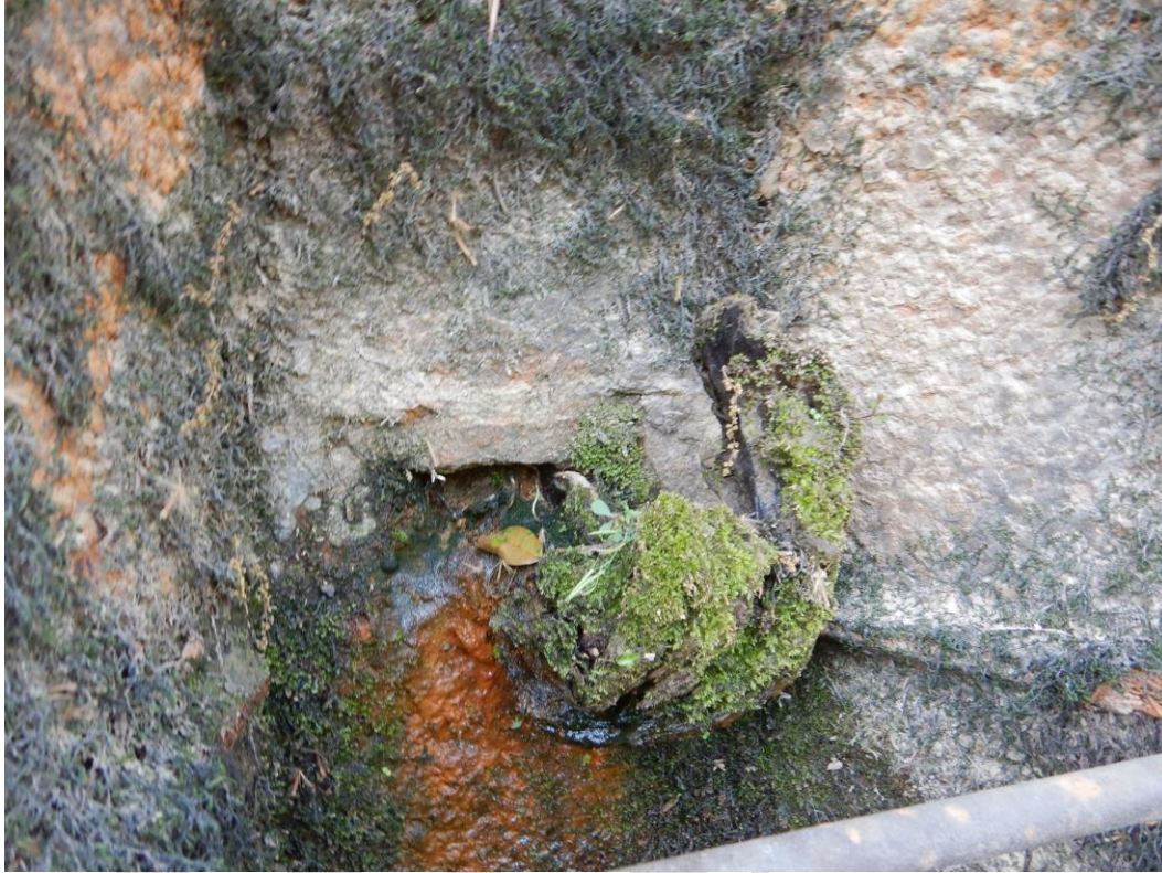
PHOTOGRAPH 2.6: TYPICAL CONDITION OF SHEET PILE WEEP HOLES
