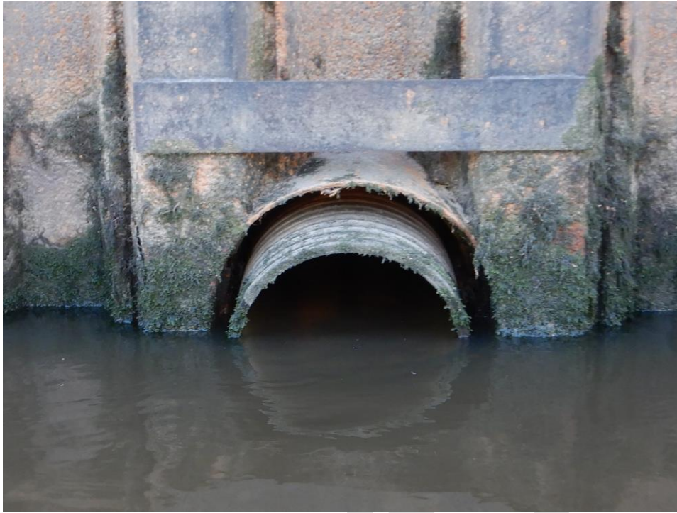
PHOTOGRAPH 2.9: CONDITION OF CMP OUTFALL AND STEEL PIPE SLEEVE AT STATION 4+18
