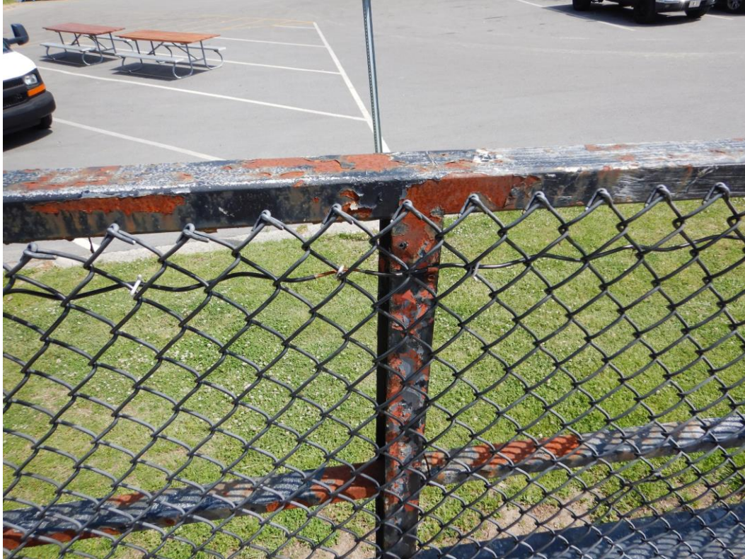
PHOTOGRAPH 2.3: TYPICAL CONDITION OF EXISTING HANDRAIL
