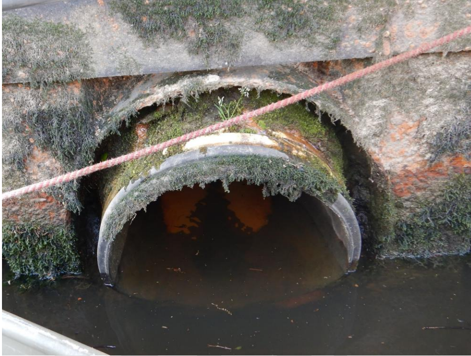
PHOTOGRAPH 2.8: CONDITION OF CMP OUTFALL AND STEEL PIPE SLEEVE AT STATION 10+38
