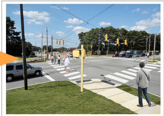
*Photo visualization showing high visibility crosswalks and pedestrian activated countdown signals.*
