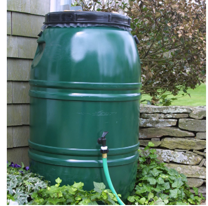
Rain barrels or cisterns can store rain water for irrigation or wash water.
