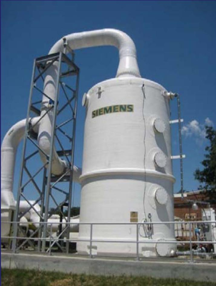
Air handling and corrosion control strategies will be implemented to address hydrogen sulfide corrosion and odors
