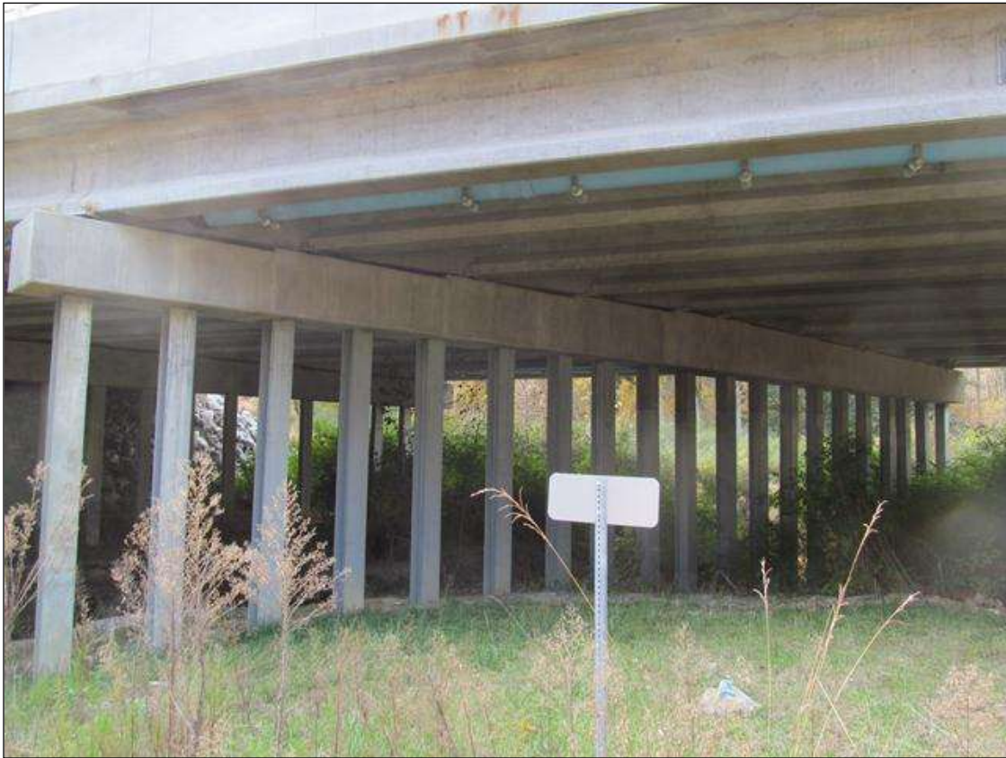
SPAN 3 SIDE OF BENT 2. (BT 2 ON PLANS)
