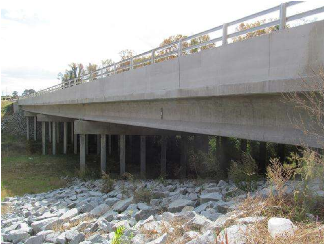
EAST SIDE, LOOKING SOUTH
