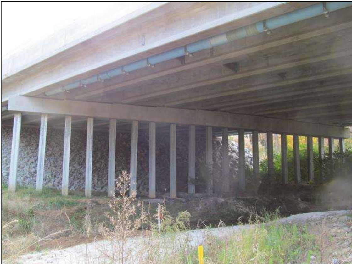
SPAN 2 SIDE OF BENT 1 (BT 3 ON PLANS)
