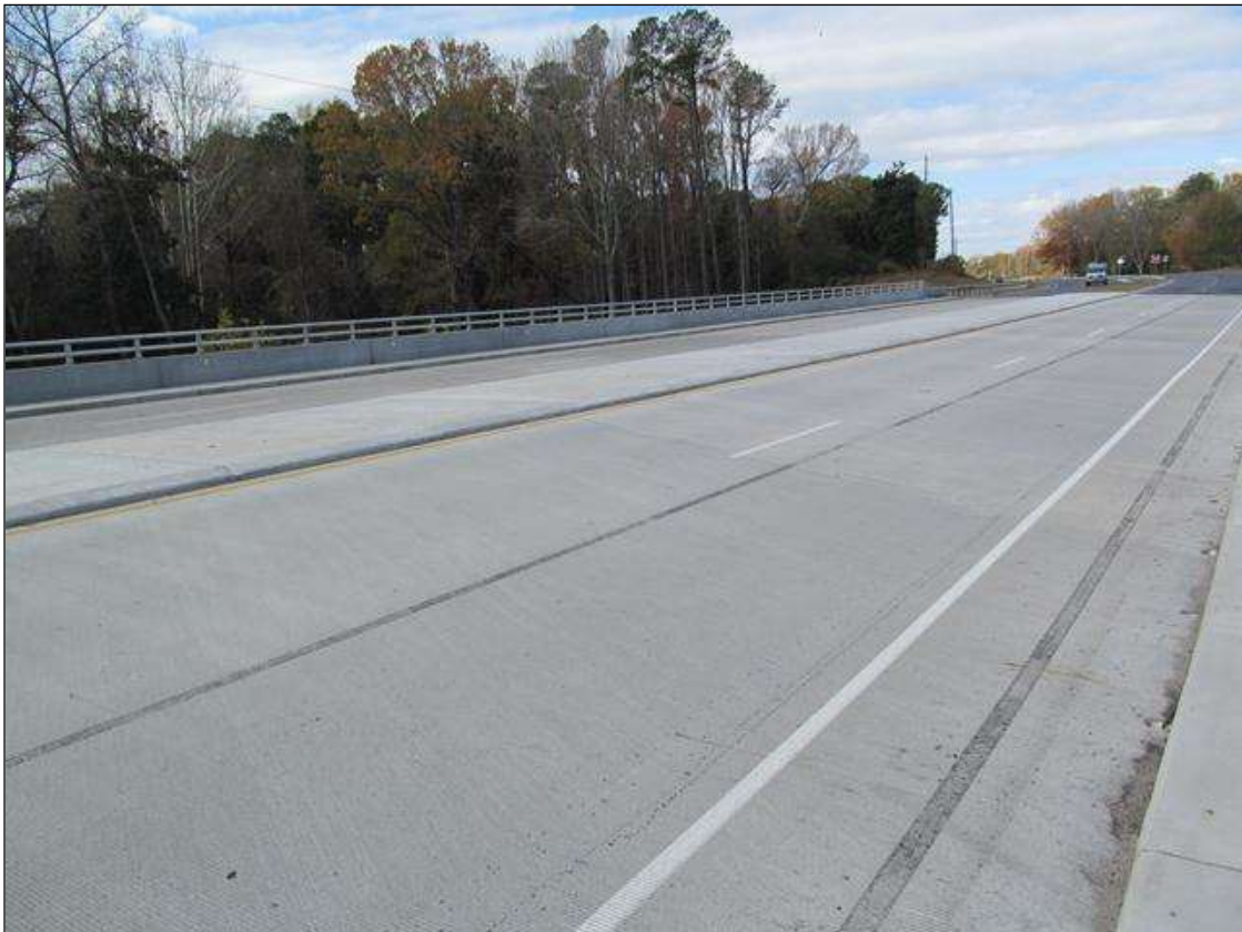
RC DECK WITH CONCRETE MEDIAN AT CENTERLINE
