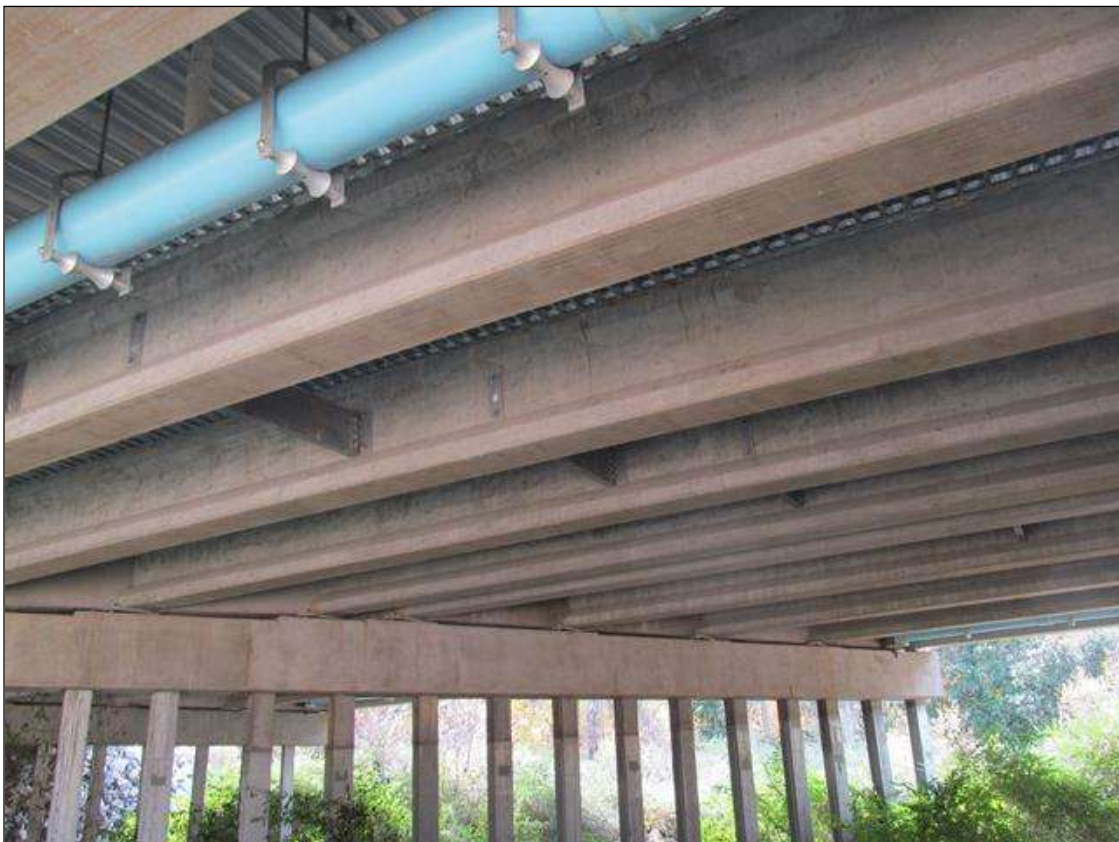
SPAN 3 UNDERSIDE. (ALL SPANS SIMILAR)
