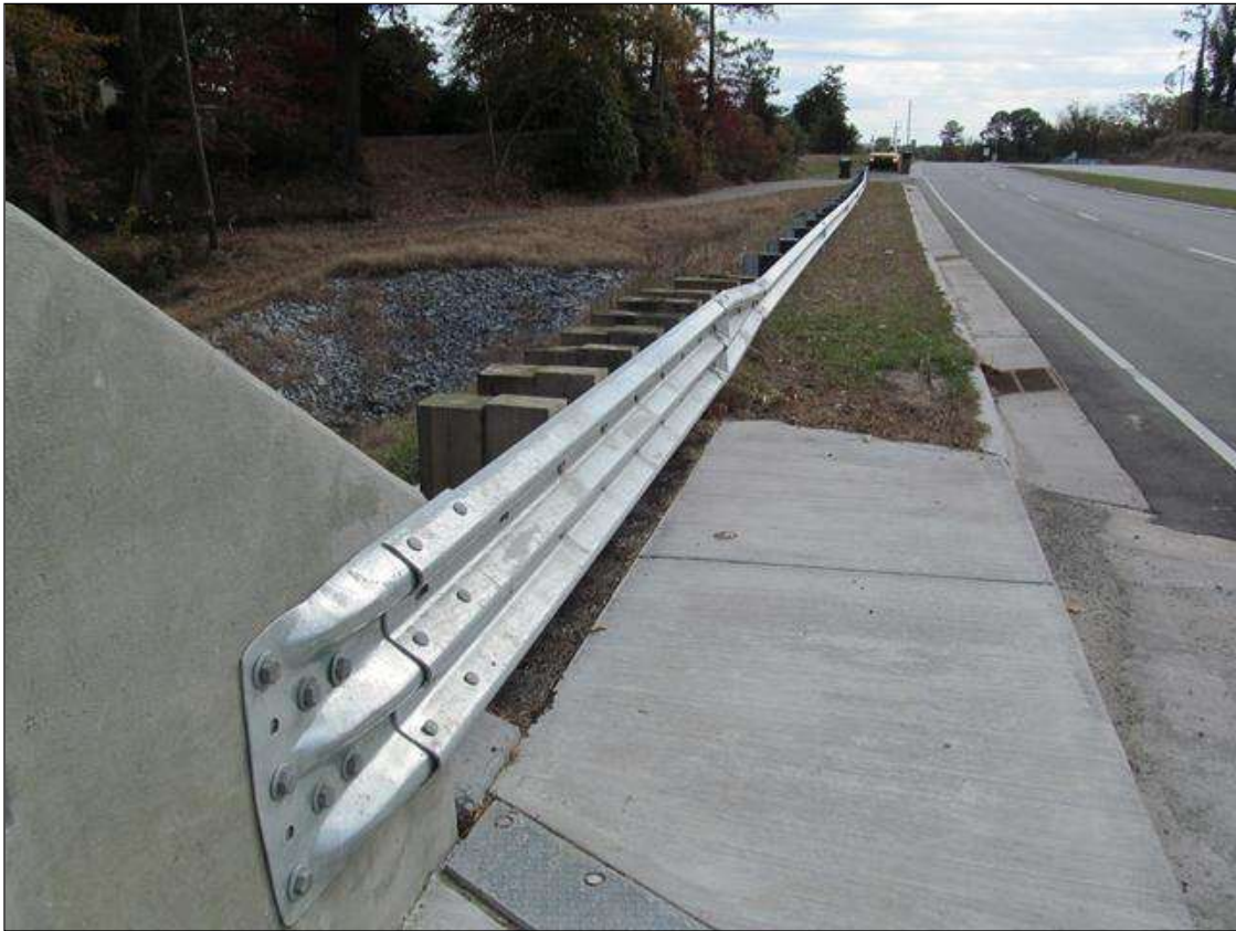
SE GUARDRAIL CONNECTION. (SE,NE,NW CONNECTIONS SIMILAR)
