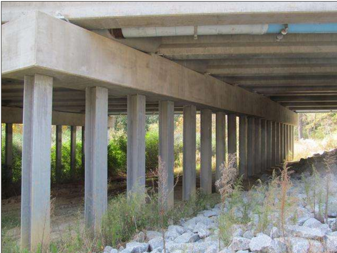
SPAN 4 SIDE OF BENT 3 (BT 1 ON PLANS)
