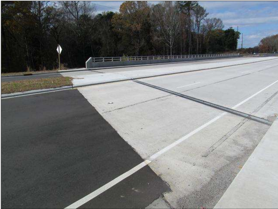
SOUTH APPROACH & SLABS. NORTH END SIMILAR.
