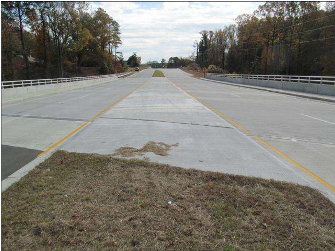
LOOKING SOUTH FROM NORTH APPROACH AT CONCRETE MEDIAN AT CENTERLINE.
