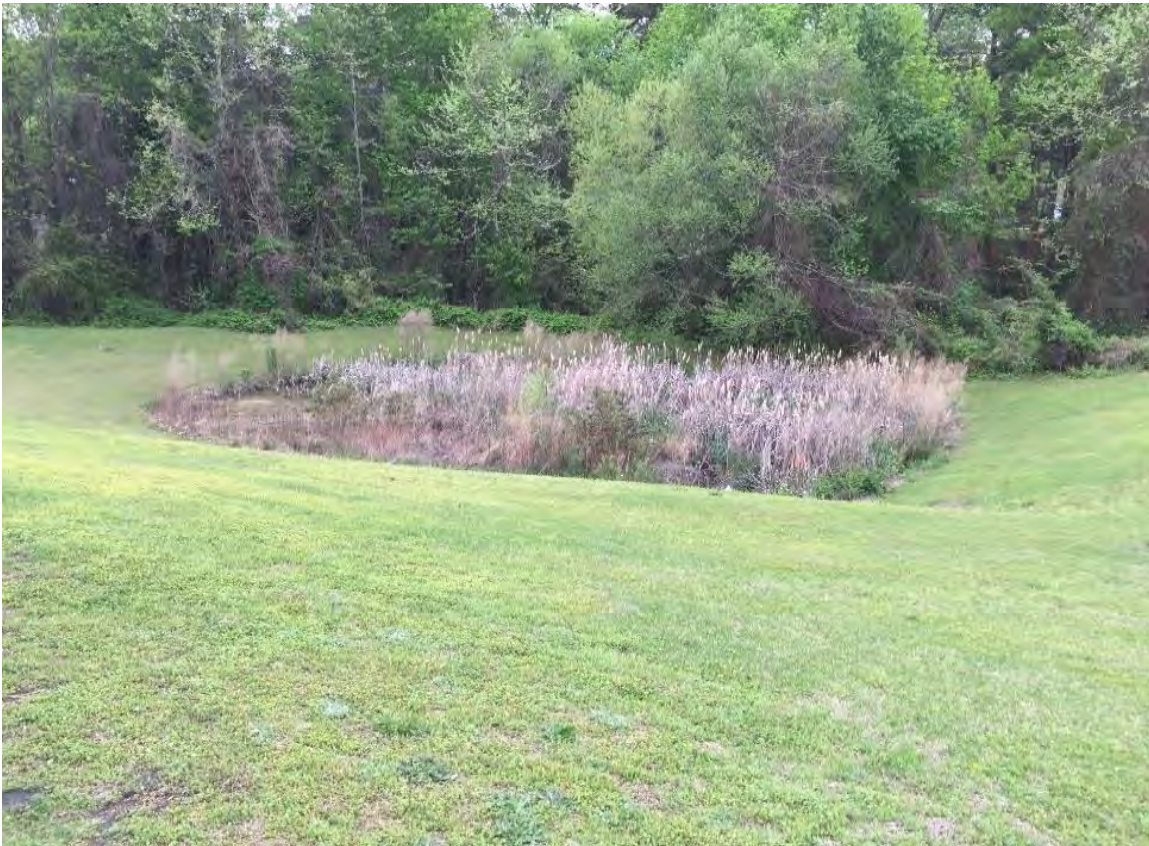
Picture 5-32: First Pentecostal Holiness Church Wet Detention Basin Retrofit
