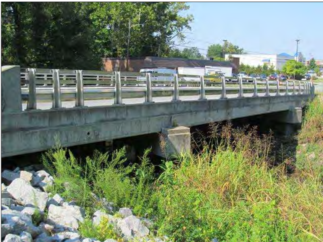
NORTH SIDE, LOOKING WEST
