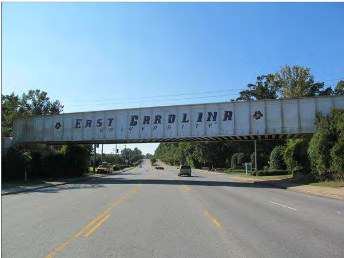
LOOKING SOUTH, SR 1707
