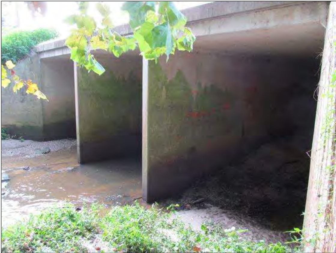
NORTH END, LOOKING EAST.
