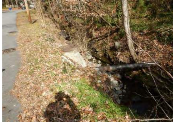
Picture 5-8: Right-of-Way on Left Floodplain and Sewer Utilities
