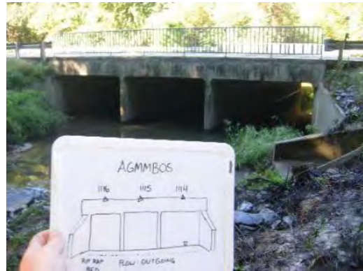
Picture H- 4. Greens Mill Run: Hooker Road Downstream Face
