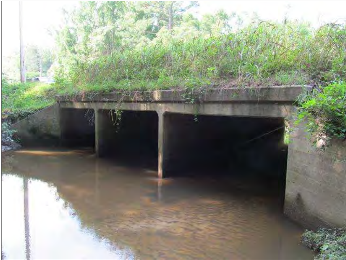
EAST END, LOOKING SOUTH
