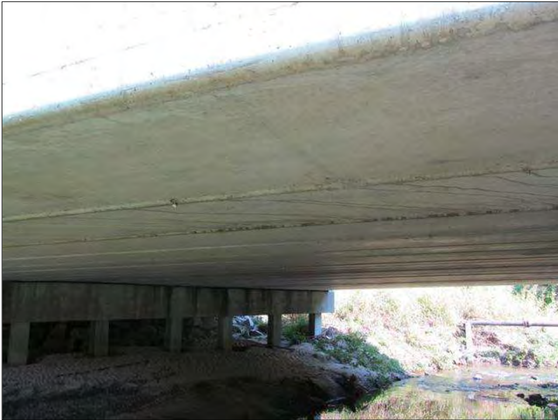
SPAN 2 UNDERSIDE. (ALL SPANS SIMILAR)
