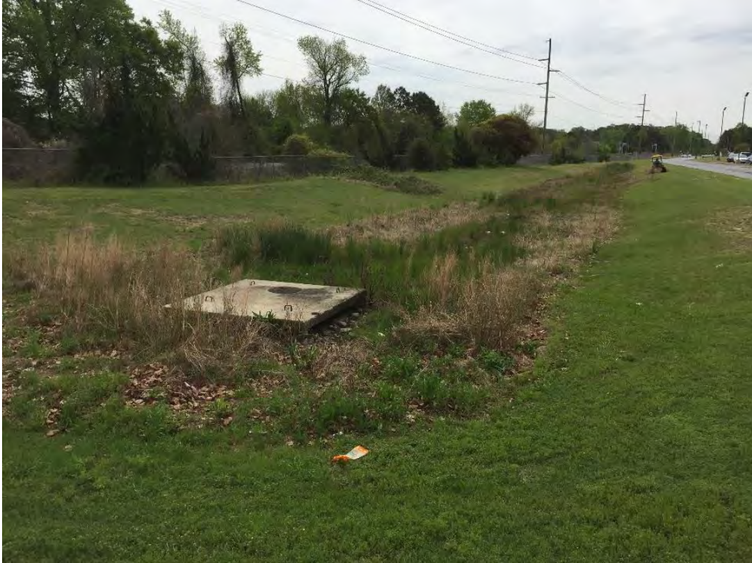
Picture 5-19: J.H. Rose High School Wet Detention Basin Retrofit
