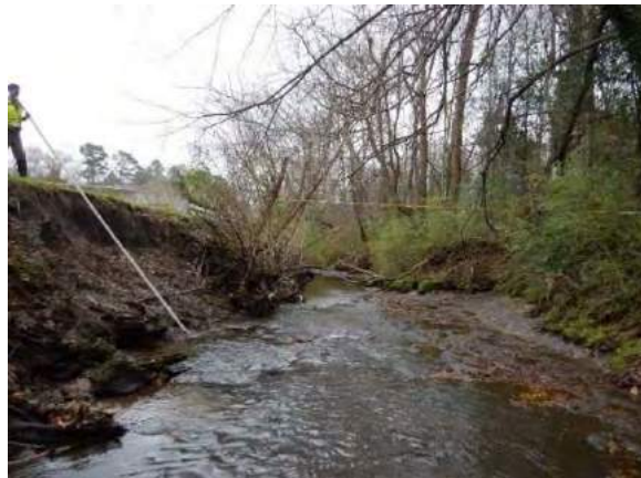
Picture 5-16: Vegetated Right Bank and Eroded Left Bank
