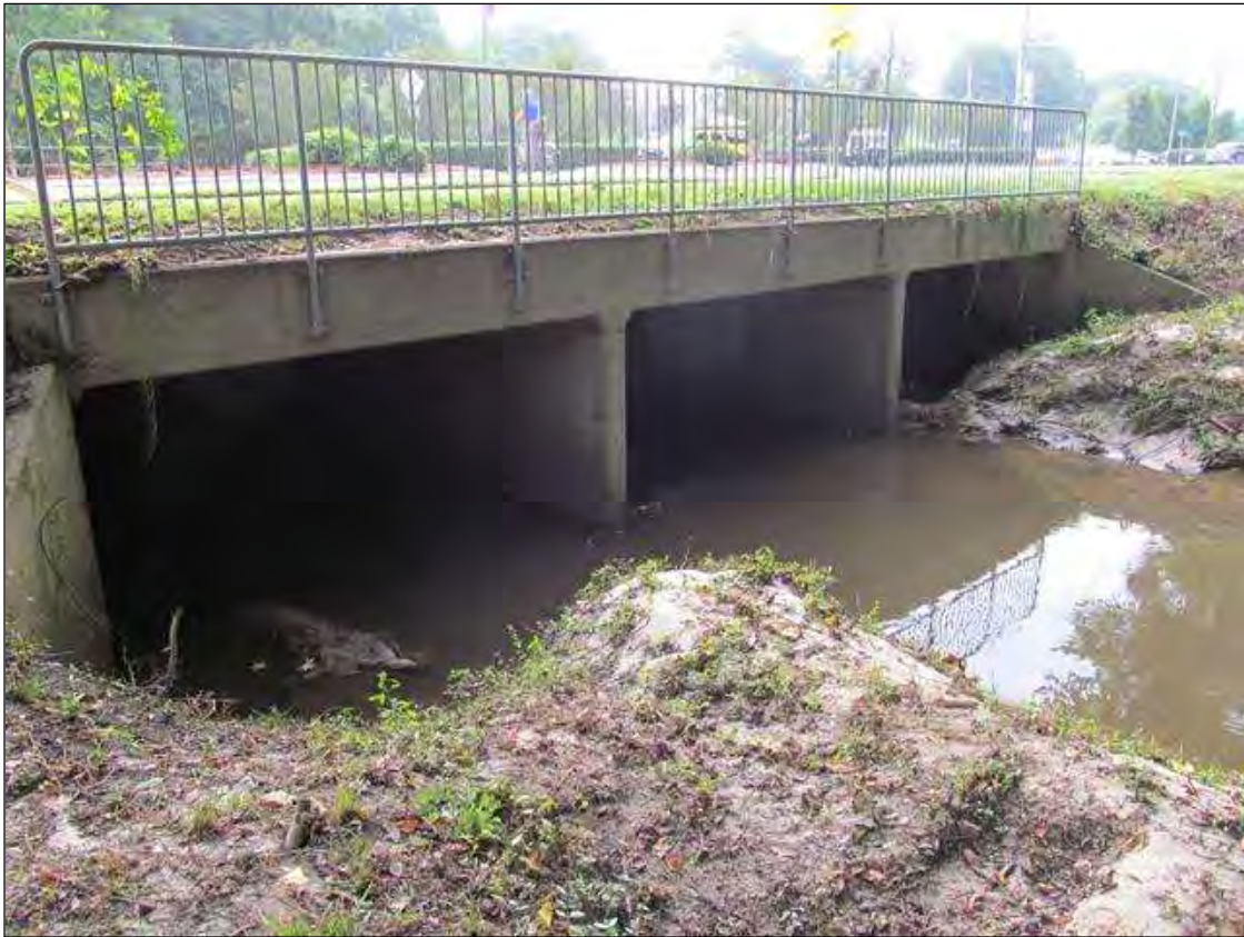
WEST END, LOOKING WEST.
