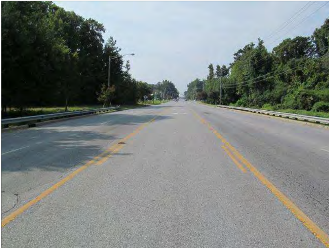
LOOKING SOUTH, SR 1702
