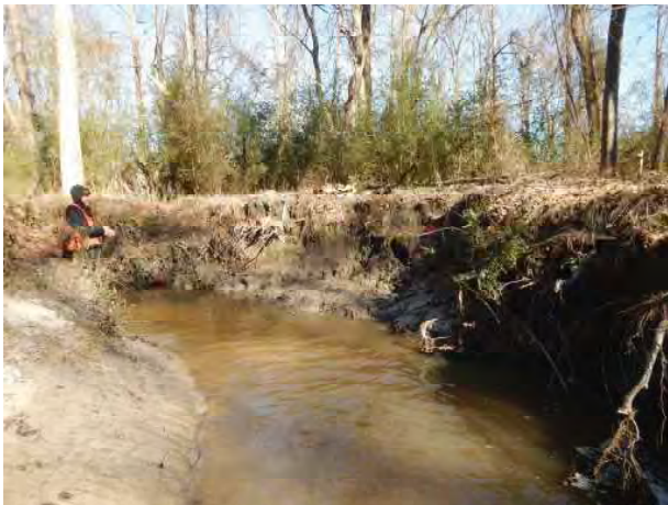
Site 1.1 Bank Pins Looking Upstream
