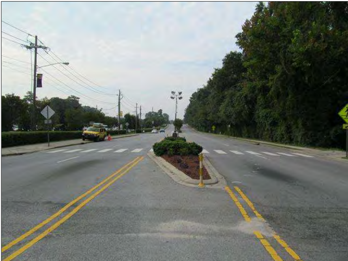
LOOKING SOUTH, SR 1707.
