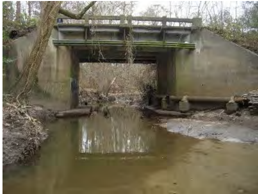
Picture H- 13. Greens Mill Run: 5th Street Upstream Face
