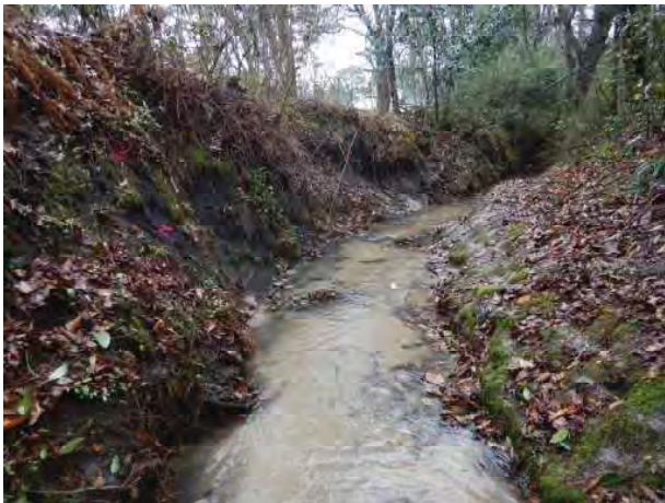
Site 11 (105 St Andrews Dr) Bank Pins Looking Downstream
