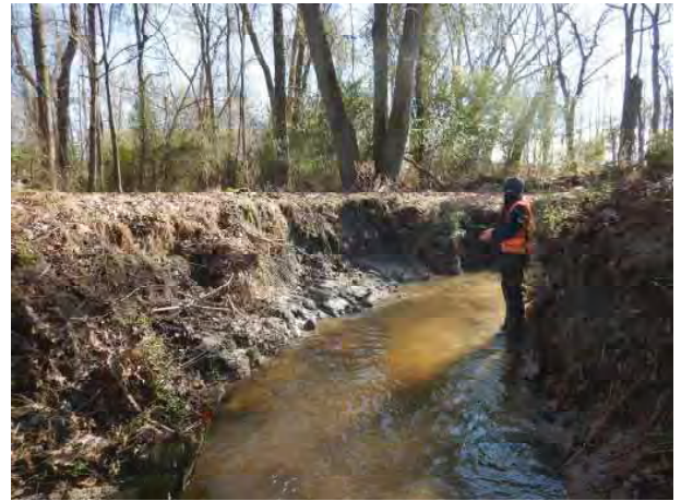
Site 1.1 Bank Pins Looking Downstream
