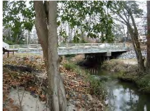
Picture H- 8. Greens Mill Run: 14th Street Upstream Face
