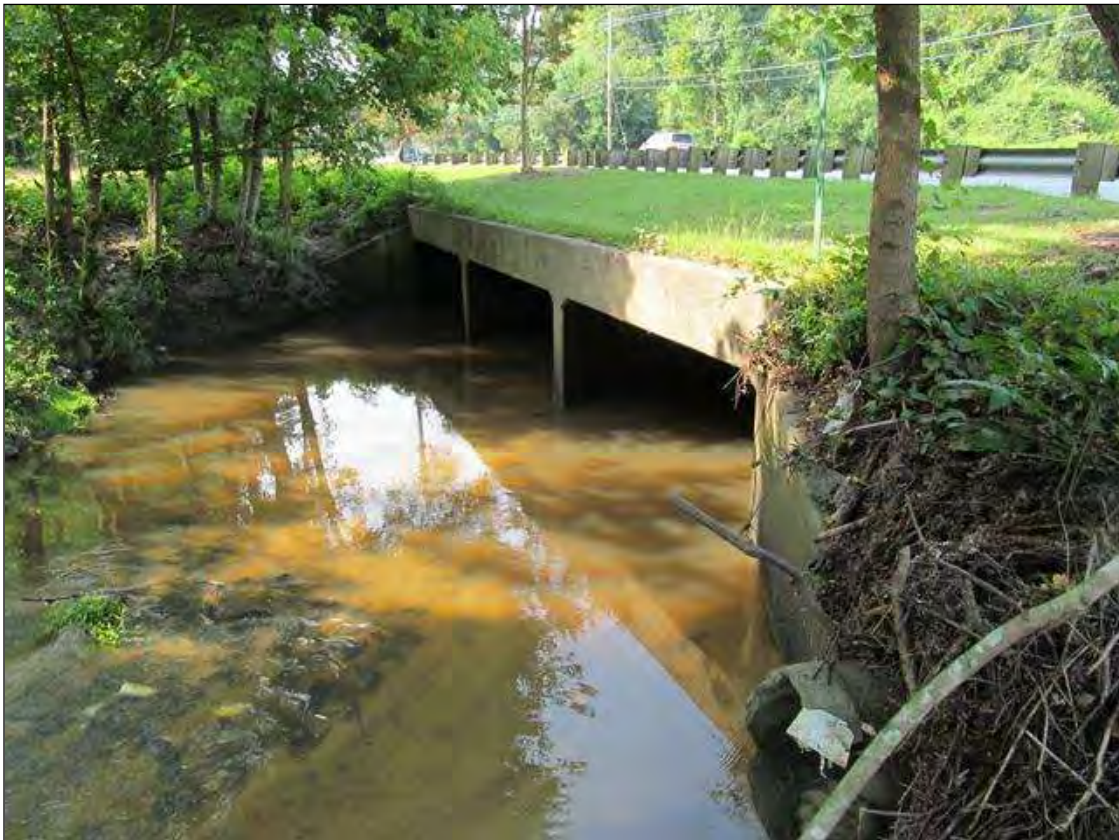
EAST SIDE, LOOKING SOUTH
