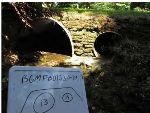
Picture H- 29. Fornes Run: Overlook Road Upstream Face
