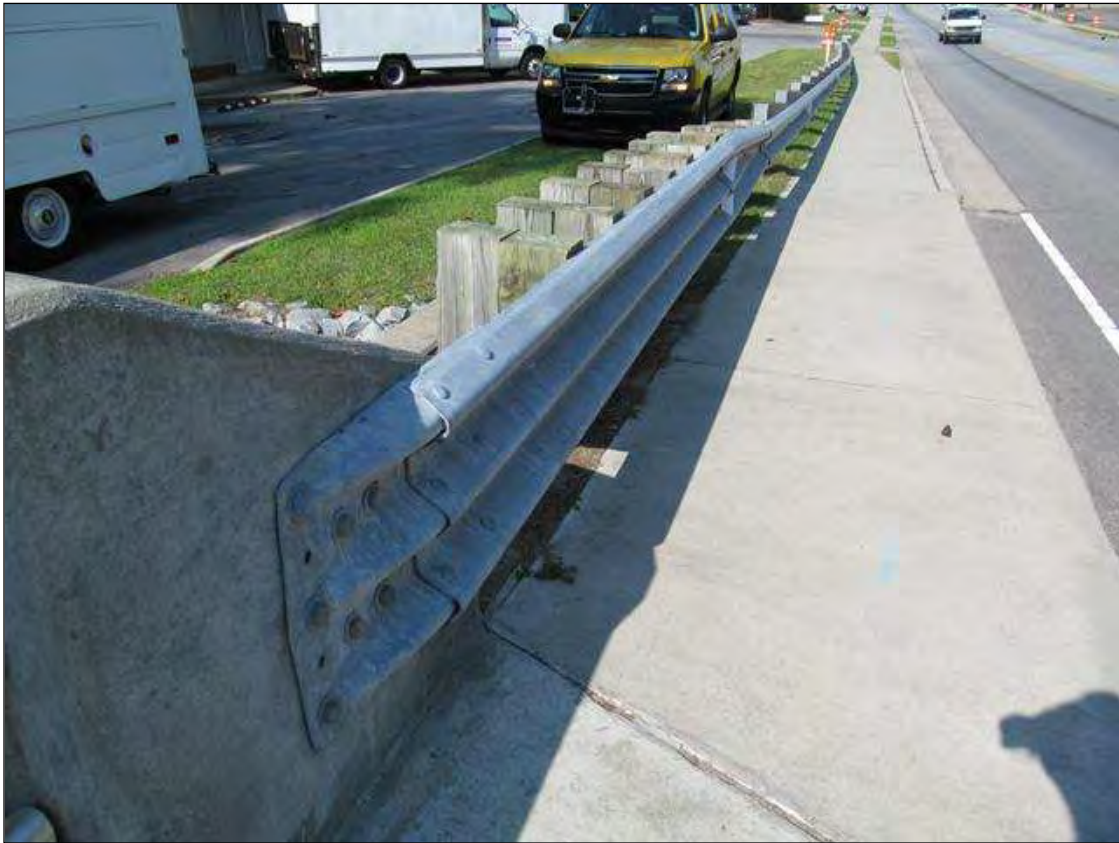
SW GUARDRAIL CONNECTION. (NE CONNECTION SIMILAR)
