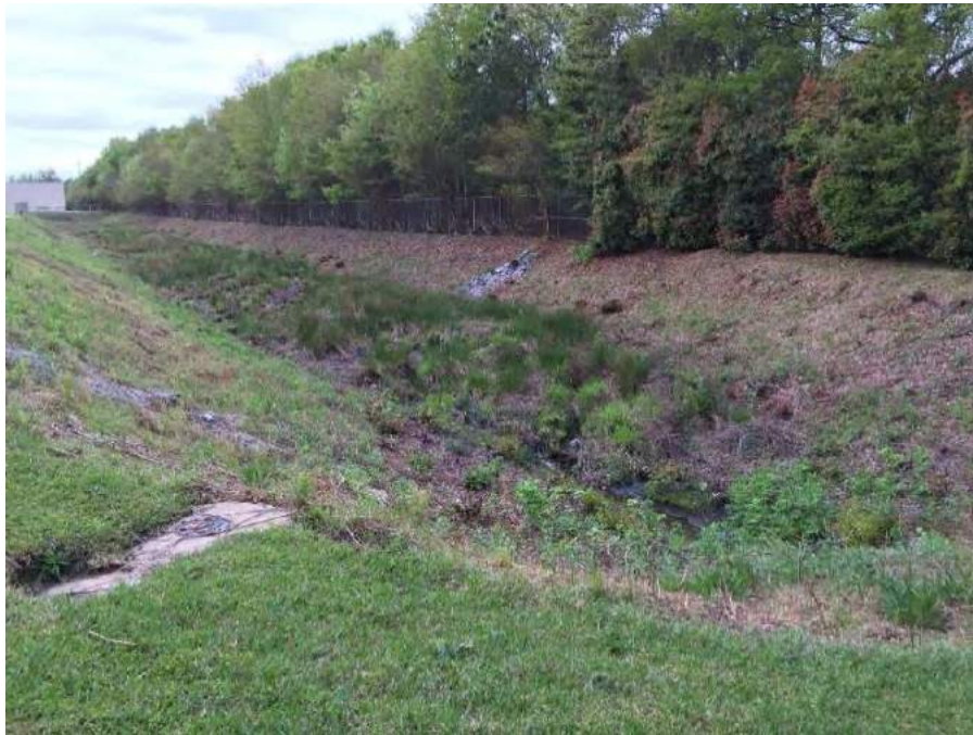
Picture 5-24: University Commons Shopping Center Wet Detention Basin Retrofit
