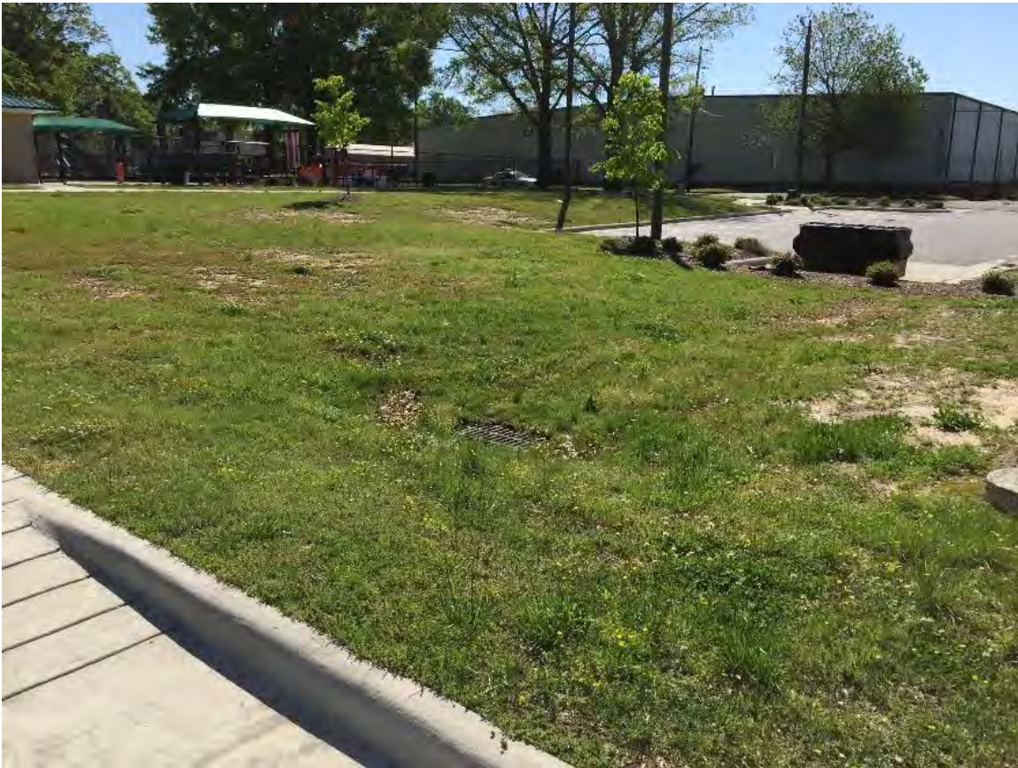
Picture 5-33: Dream Park Bioretention Area
