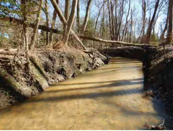
Site 4.2 Bank Pins Looking Downstream
