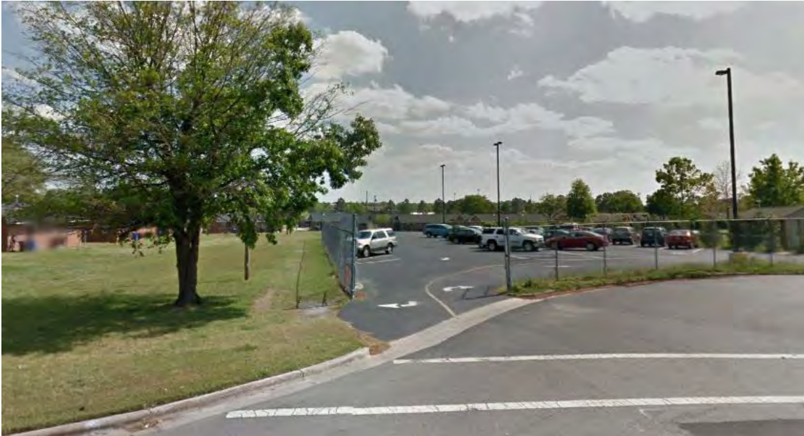
Picture 5-26: South Greenville Elementary School Bioretention Area
