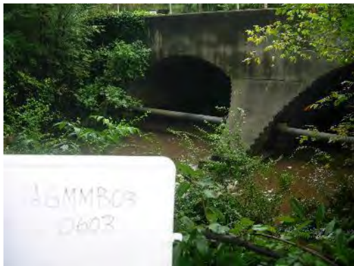
Picture H- 11. Greens Mill Run: Elm Street Downstream Face
