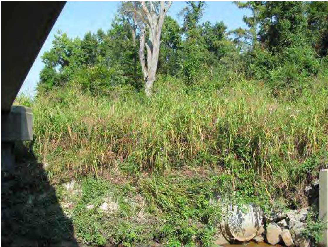
VEGETATION AT NW SLOPE. SIMLAR AT NE & SW SLOPES.
