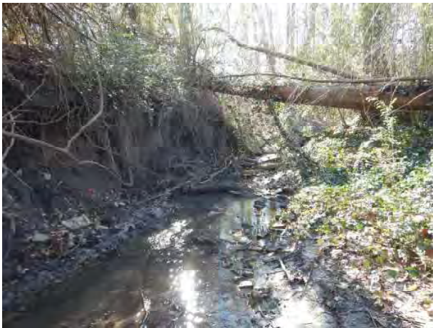
Site 9.1 Bank Pins Looking Upstream
