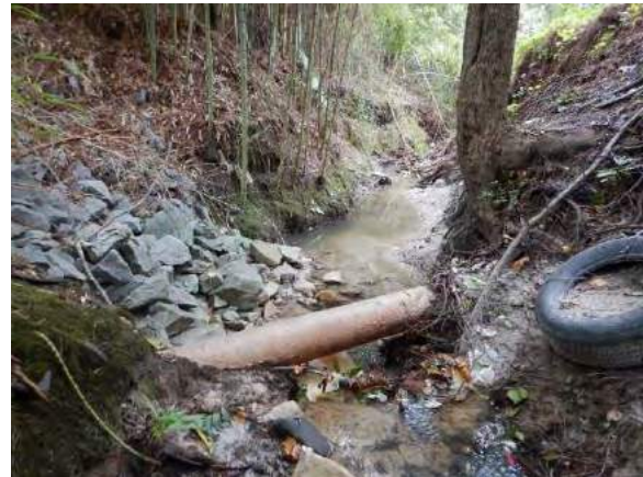
Picture 5-11: Exposed Gravity Sewer Crossing
