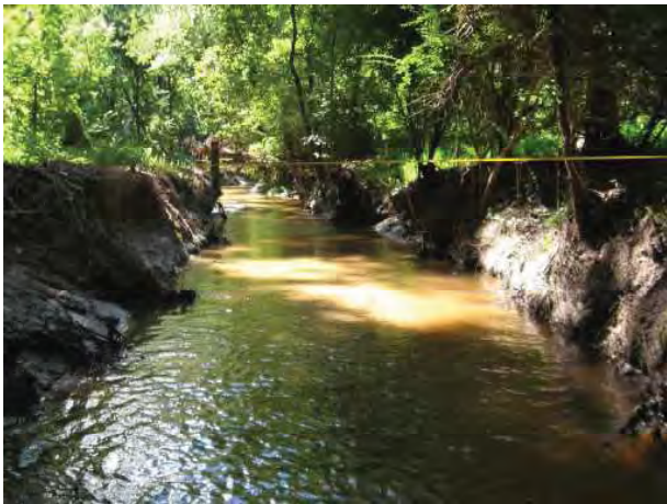
BEHI 4.2 Looking Upstream at XS 4.2
