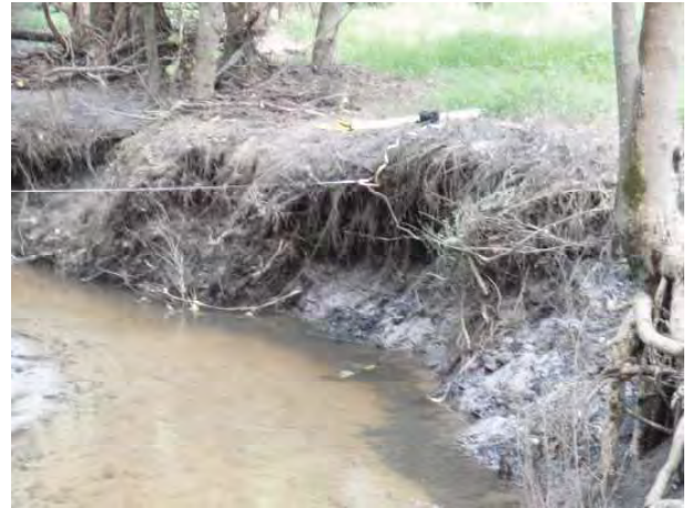
BEHI 4.1 Looking Downstream at XS 4.1
