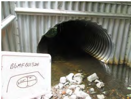
Picture H- 33. Fornes Run: Dalebrook Circle Upstream Face
