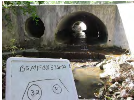
Picture H- 28. Fornes Run: Crestwood Drive Downstream Face
