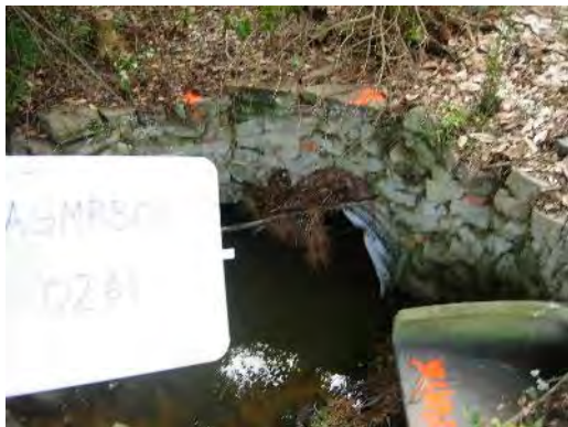
Picture H- 35. Reedy Branch: Greenville Boulevard Upstream Face
