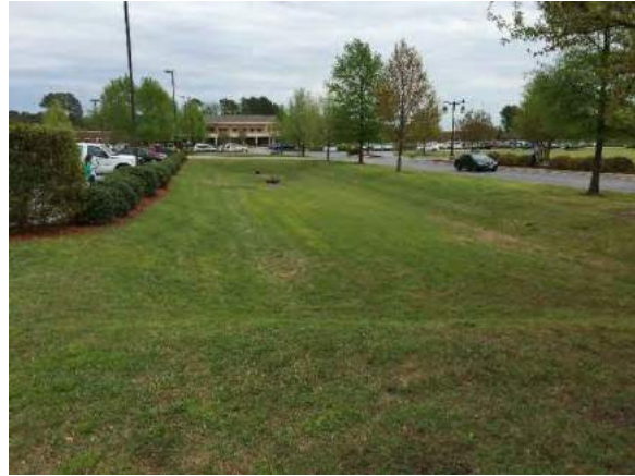
Picture 5-36: Arlington Crossing Shopping Center Wet Detention Basin Retrofit (South)
