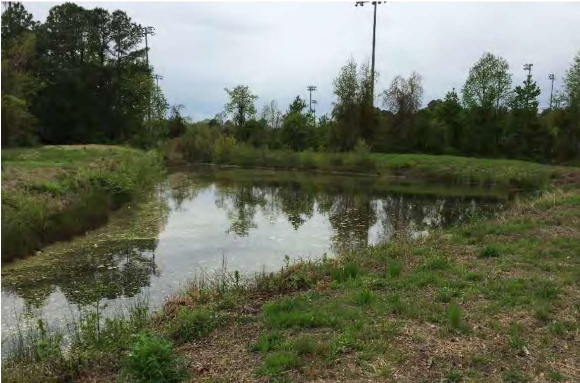
Picture 5-21: Greenville Square Shopping Center Wet Detention Basin Retrofit
