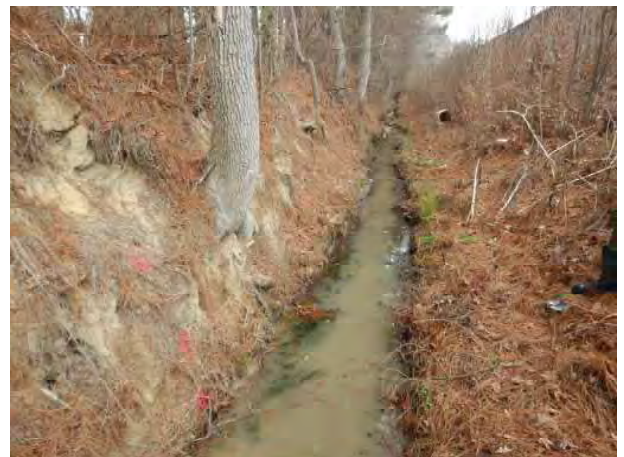
Site 11 (403 St Andrews Dr) Bank Pins Looking Downstream
