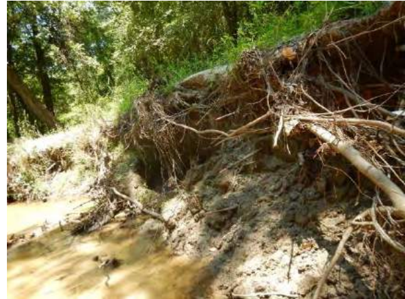
Picture 5-2: Stream Bank and Pins Five Months Later
