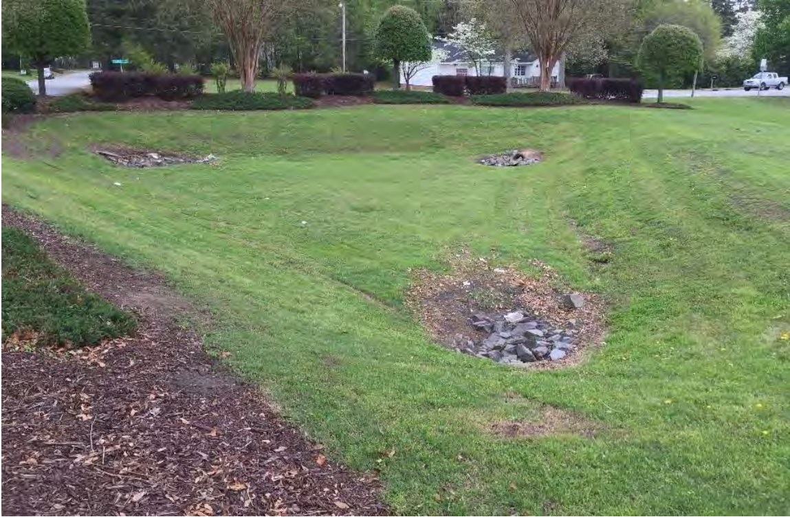
Picture 5-22: Pirates Pointe Shopping Center Wet Detention Basin Retrofit
