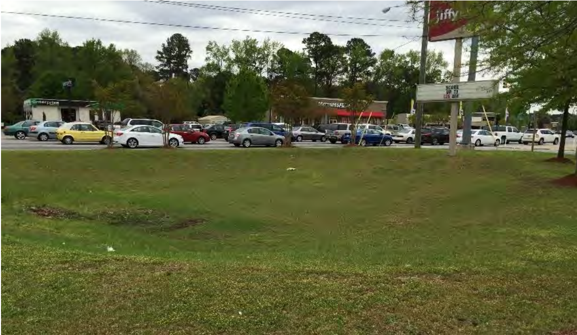
Picture 5-29: Jiffy Lube Bioretention Area Retrofit
