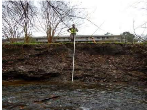
Picture 5-15: Left Bank Erosion
