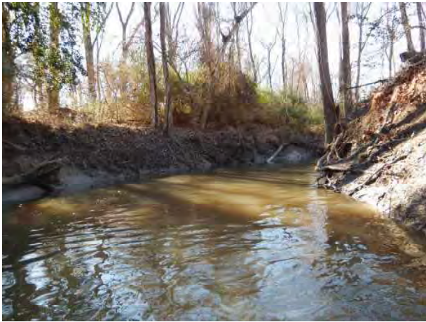
Site 10.3 Bank Pins Looking Upstream
