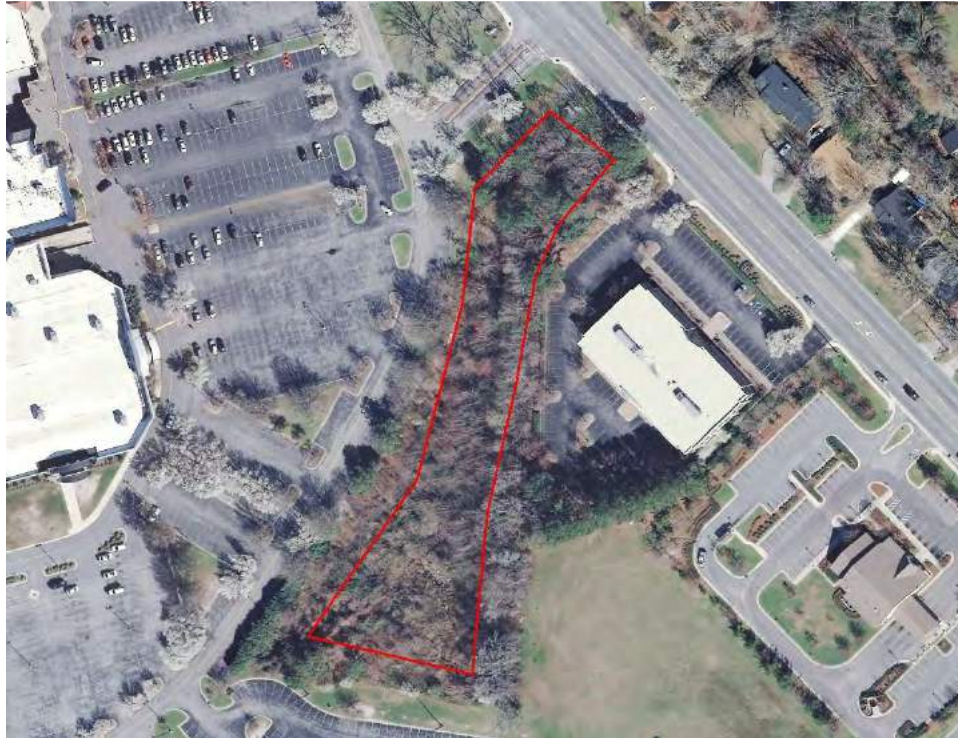
Picture 5-23: Greenville Mall Wet Detention Basin Retrofit
