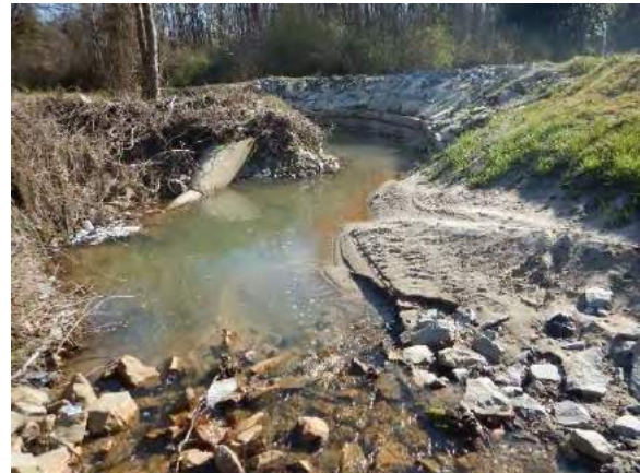
Picture 5-9: Existing Imbricated Riprap Wall on Right Bank
