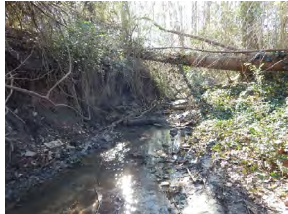
Picture 5-5: Right Stream Bank Erosion
