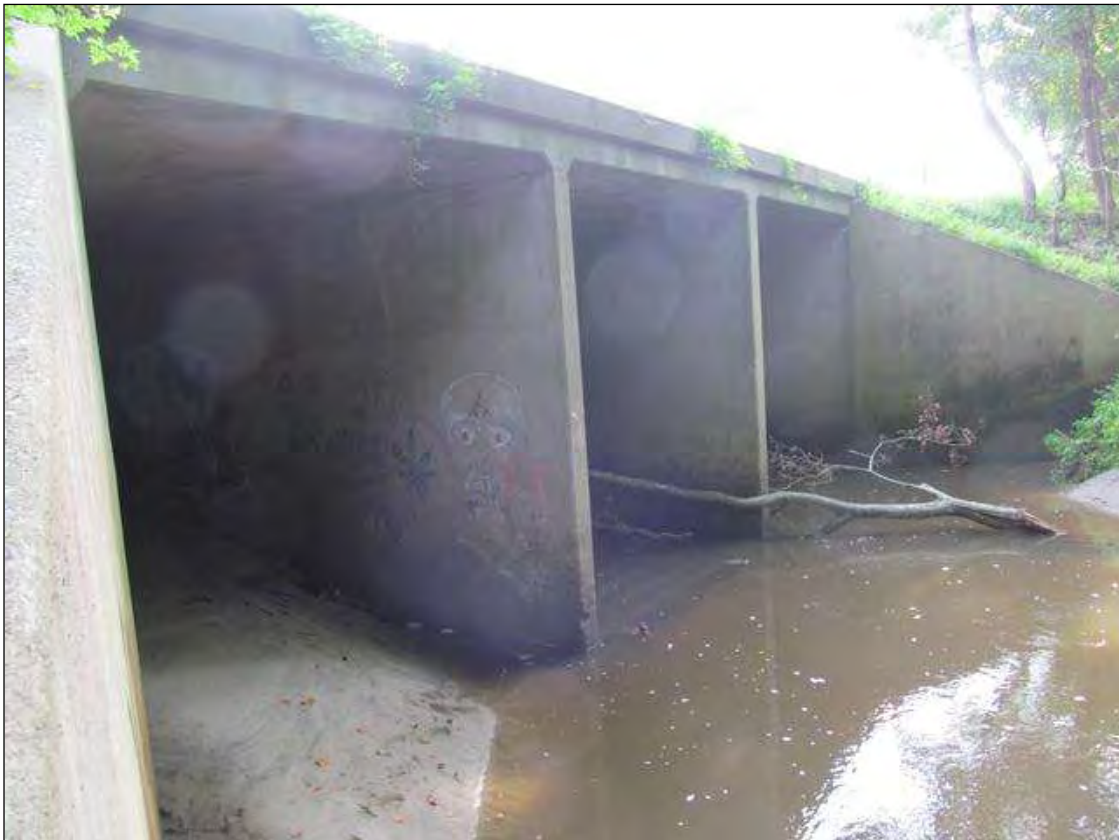
SOUTH END, LOOKING EAST.
