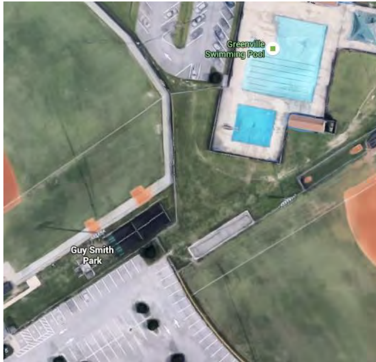
Picture 5-25: Guy Smith Park Bioretention Area
