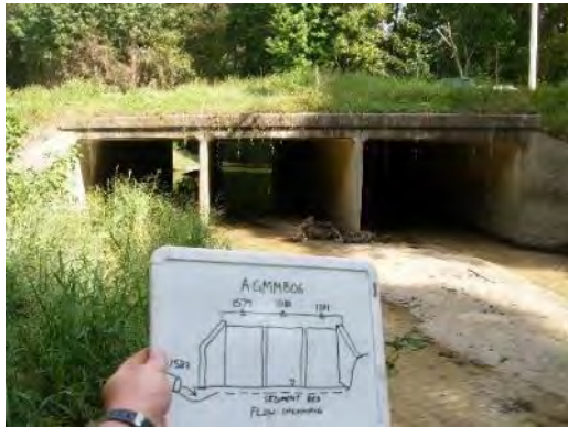
Picture H- 3. Greens Mill Run: Memorial Drive Upstream Face
