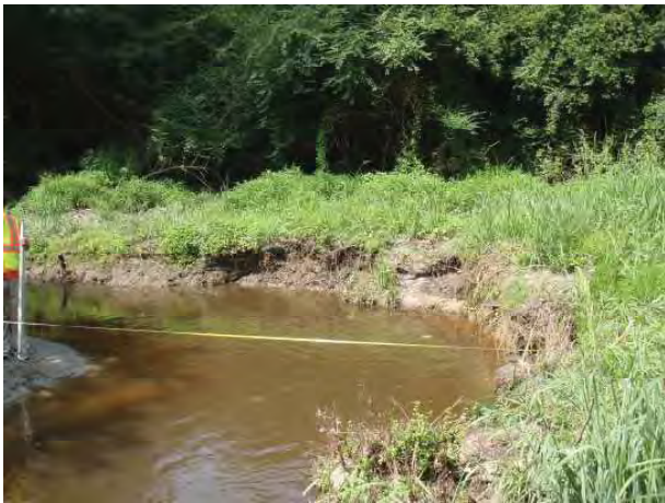
BEHI 6.1 Looking Upstream at XS 6.1
