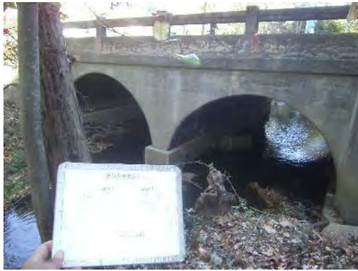
Picture H- 9. Greens Mill Run: Rock Spring Road Upstream Face
