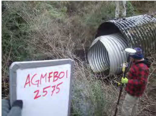
Picture H- 31. Fornes Run: Railroad Downstream Face
