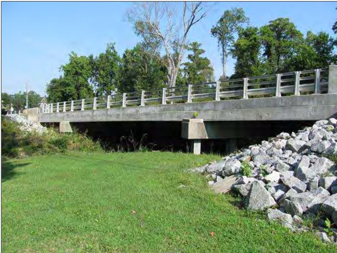
SOUTH SIDE, LOOKING WEST
