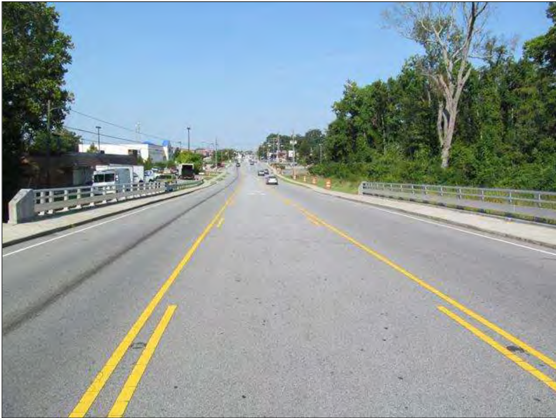
LOOKING WEST, SR 1703
