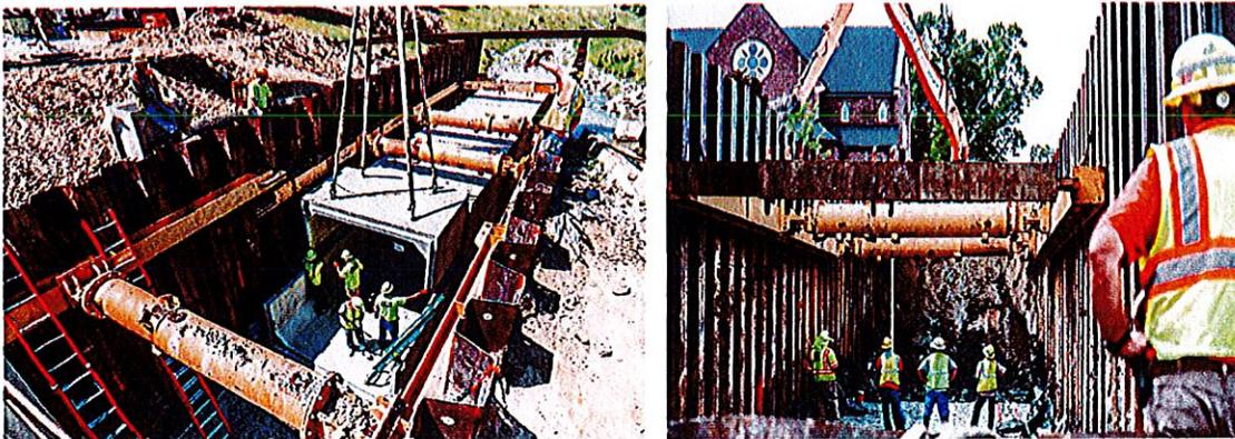
Once the 3<sup>rd</sup> Street RCBC was placed, Trader Construction began removing the existing arch culvert between 3<sup>rd</sup> Street and 4<sup>th</sup> Street making the new RCBC live and operational.
