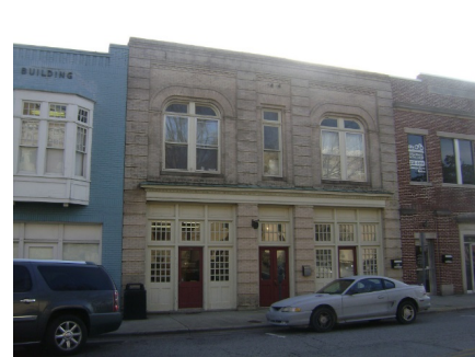
105-107 West Third Street Hassel - James Building & Grounds
