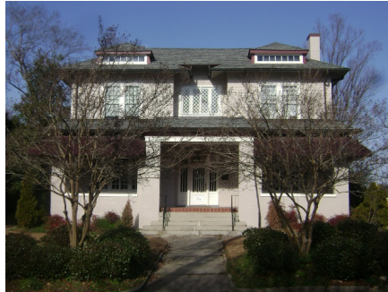
402 West Fourth Street Alfred M. Moseley House & Grounds
