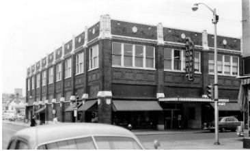
330 Evans Street Blount Harvey Building
