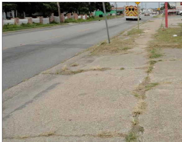
Some sidewalk are cracked, overgrown and/or are no longer level. Above: Sidewalk on Dickinson Avenue.
