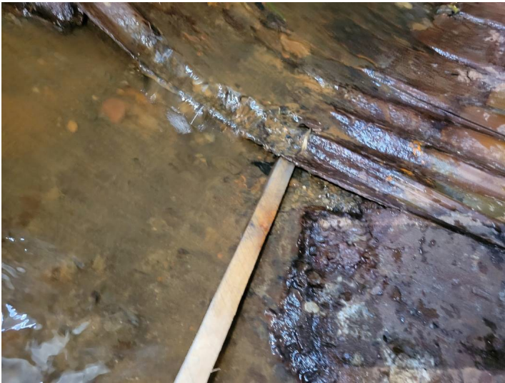
Photo 10 At MH base, erosion under pipe, sta 1+90
