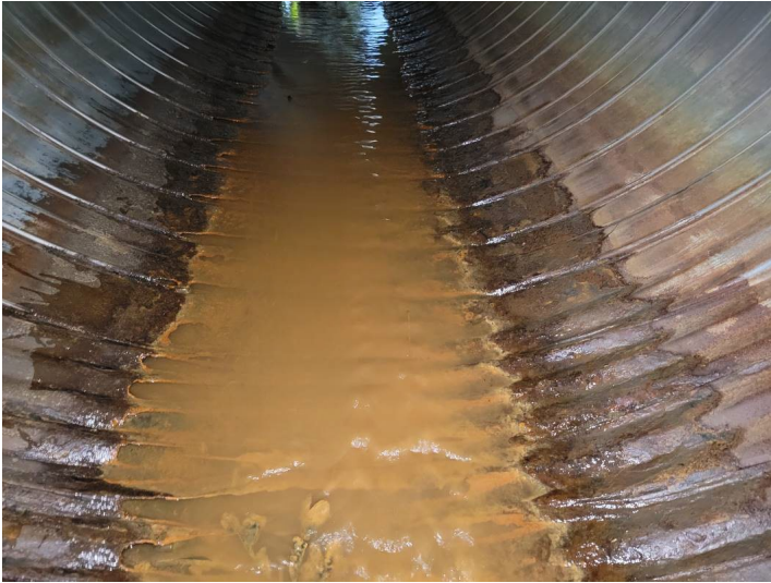
Photo 31 Sta 14+10 Severe corrosion with penetrations
