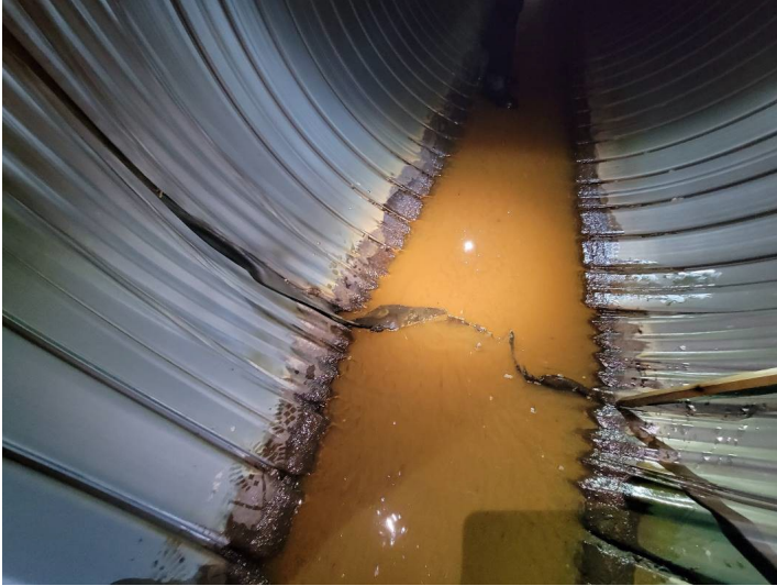
Photo 19 Sta 6+82, severe corrosion with gasket displaced
