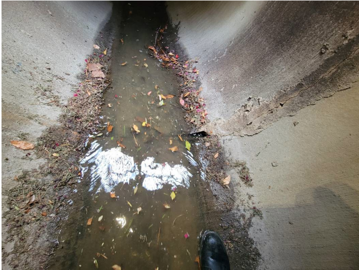
Photo 3 Water level in RCP. Note deteriorating joint
