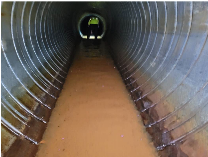
Photo 38 Sta 18+00 Minor corrosion. Smell of diesel
