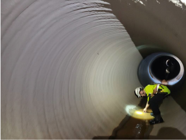
Photo 21 Spray liner from sta 7+33 to 7+61
