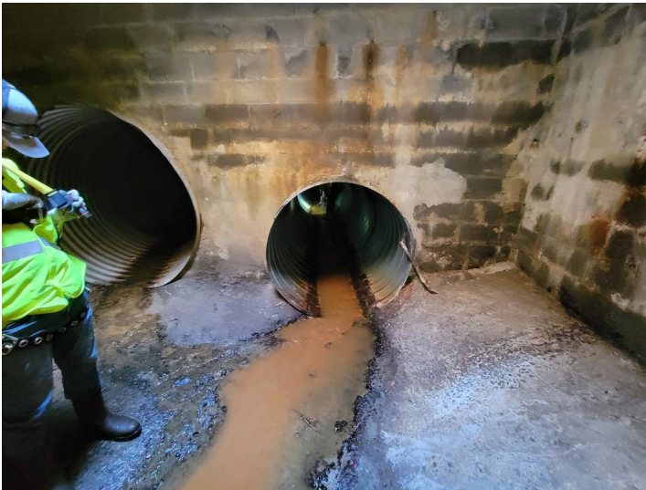
Photo 34 Sta 15+54 Manhole with second 84" entrance, 54" exit (presumed to be at or near railroad)
