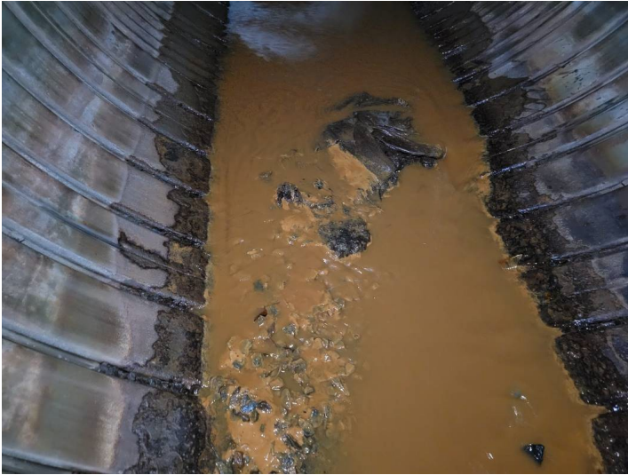
Photo 33 Sta 14+62 Significant sediment and debris
