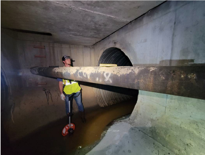
Photo 15 Sta 4+88 Manhole with water line
