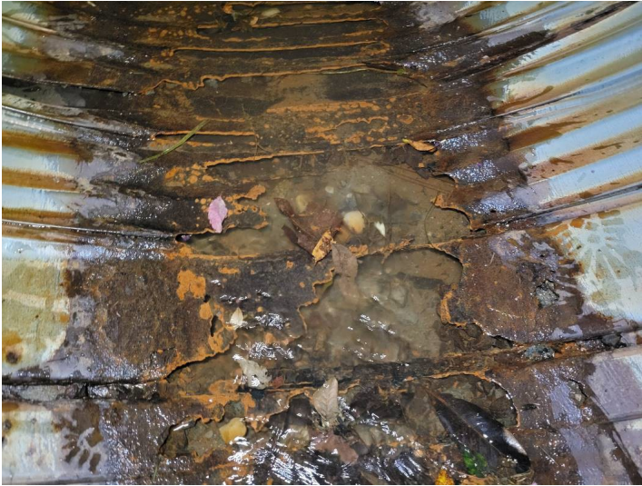
Photo 9 CSP below water line, typ sta 0 to 1+90
