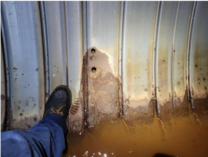
Photo 16 Sta 4+94 Severe corrosion breaching the pipe with visual evidence of soil erosion
