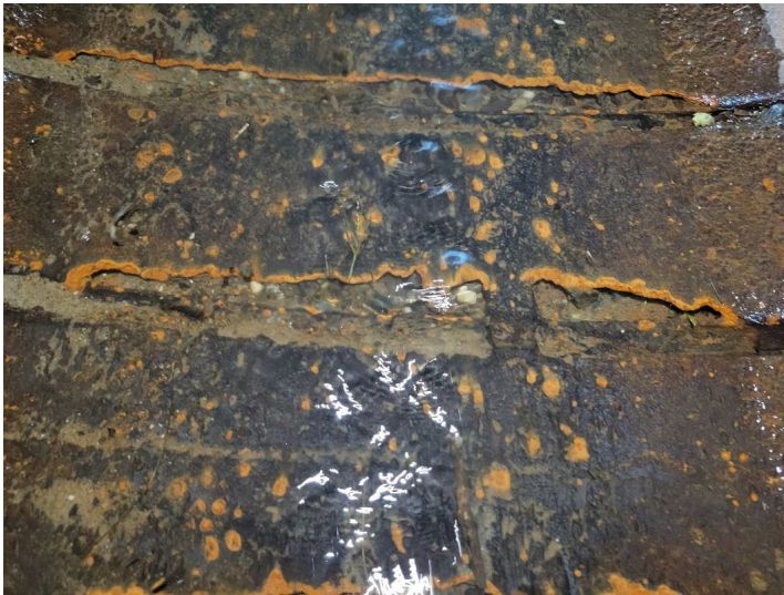
Photo 8 CSP below water line, typ sta 0 to 1+90
