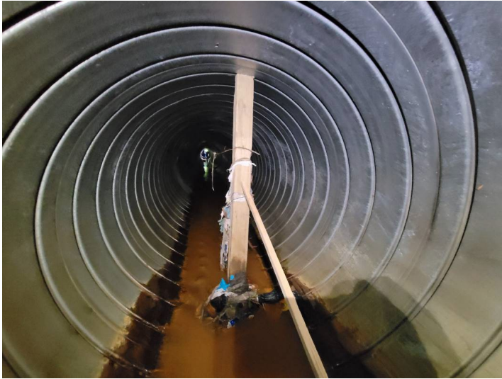
Photo 35 Sta 15+75 4x4 post in 54" pipe
