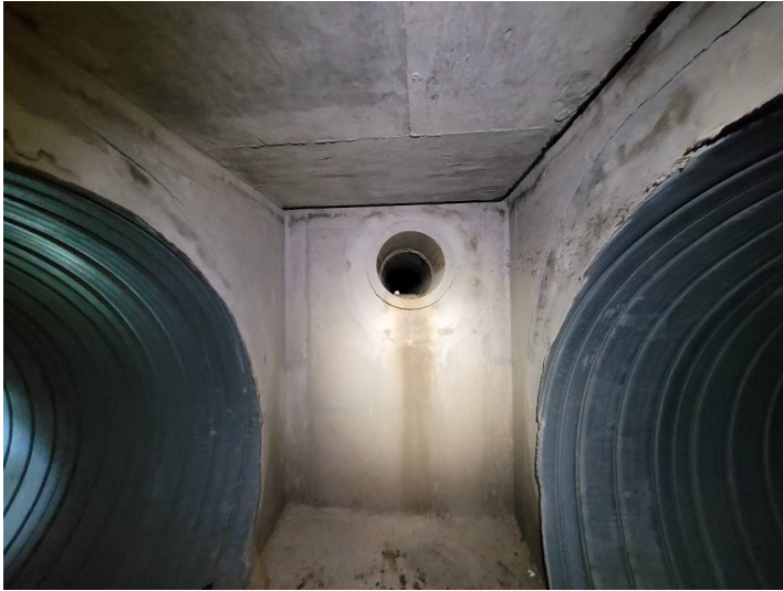
Photo 17 Sta 6+00 Manhole with 24" lateral
