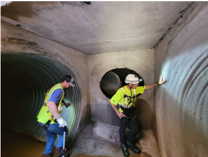
Photo 20 Sta 7+33 Manhole at spray liner trial
