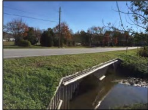
Figure 5. Corey Rd CMP arches
