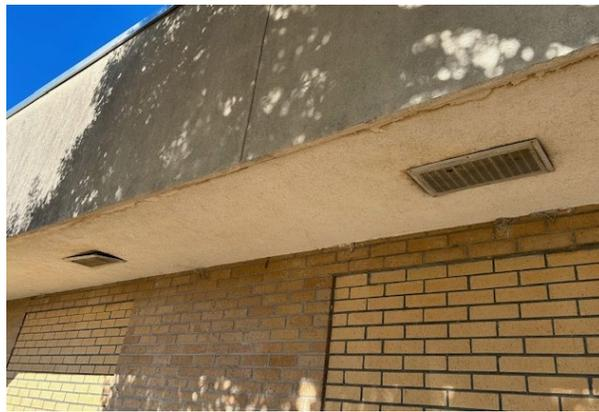
At the right rear of the gym, cover the exposed plywood on the soffit with metal and paint to match existing soffit as close as possible.
