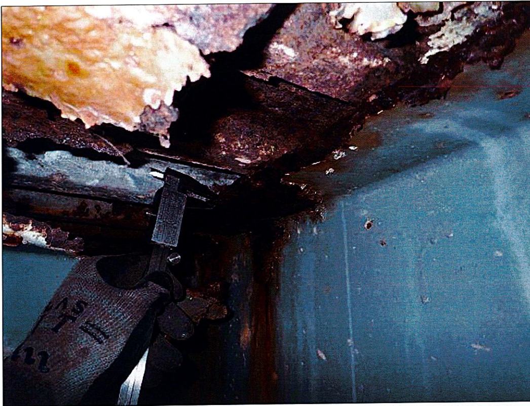
Span 1 Beam 2: 5 FEET OF RUST SCALE IN TOP FLANGE AT END BENT 2 WITH 3/16 INCHES REMAINING IN THE TOP FLANGE. (MUNICIPAL PAR)
