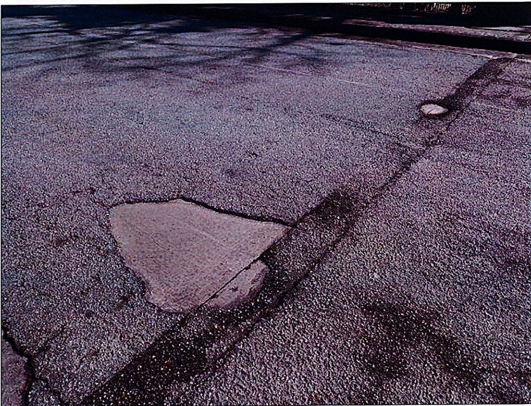
Span 1 Wearing Surface: THREE AREAS OF MISSING ASPHALT WEARING SURFACE AT END BENT 1.
