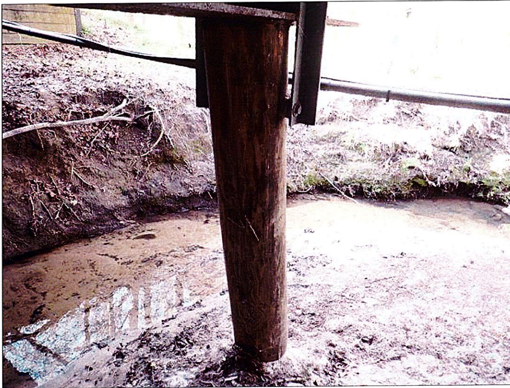
Bent 1 Pile 1: FULL HEIGHT CHECKS UP TO 5 INCHES DEEP.
