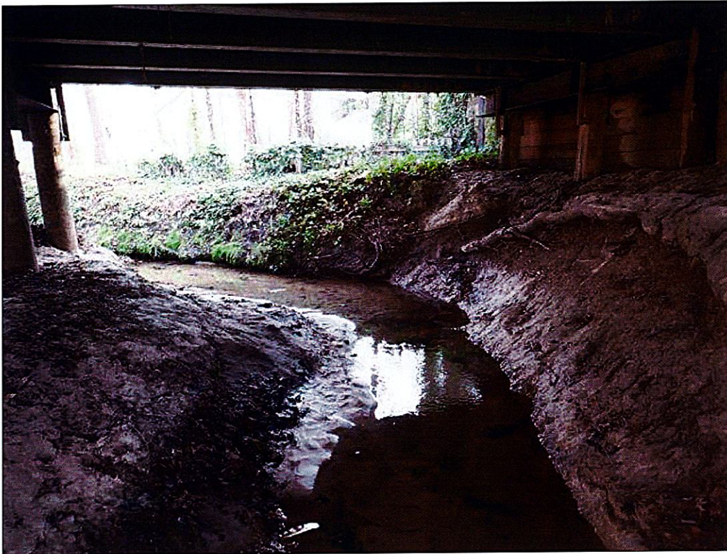
STREAMBANK NEAR END BENT 1 HAS 6 FEET TALL VERTICAL BANKS. WEST BANK HAS ERODED TO WITHIN 2 FEET OF END BENT 1 PILES
