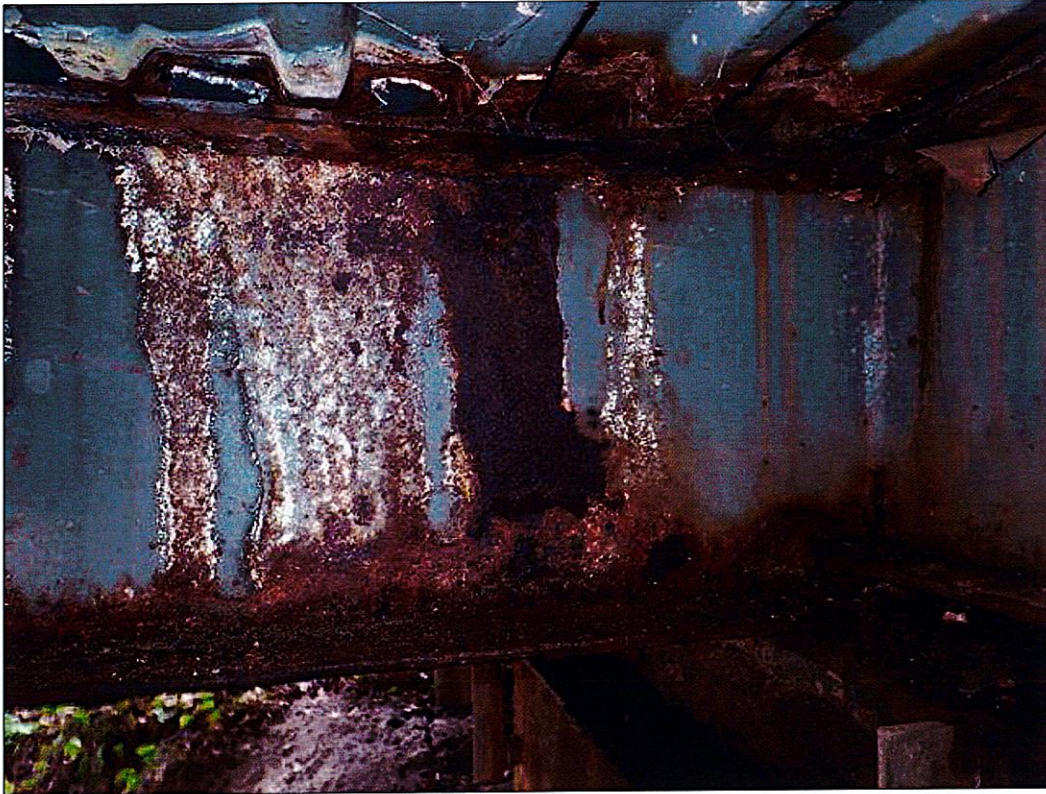
Span 1 Beam 6: 4 FEET OF RUST SCALE IN TOP AND BOTTOM FLANGES AND UP TO FULL HEIGHT IN THE WEB AT END BENT 1 WITH 3/16 INCHES REMAINING IN THE BOTTOM FLANGE, 1/4 INCHES REMAINING IN THE TOP FLANGE, AND NO MEASURABLE SECTION LOSS IN THE WEB. (MUNICIPAL PAR)
