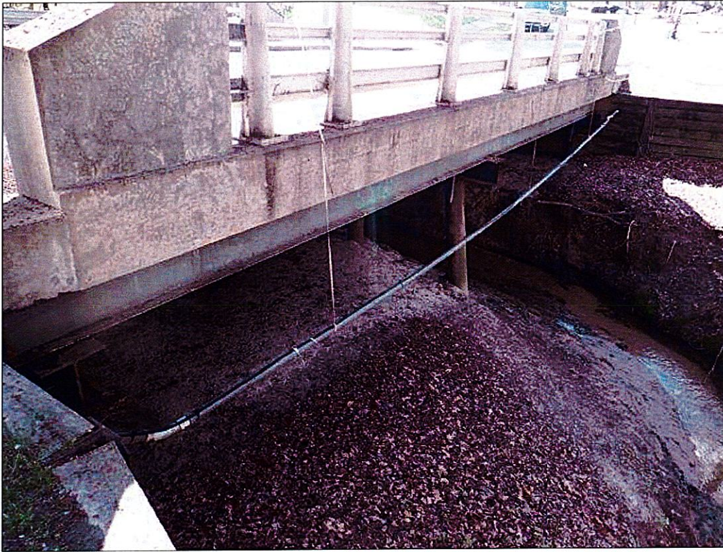
3 INCH DIAMETER UTILITY AT NORTH END
