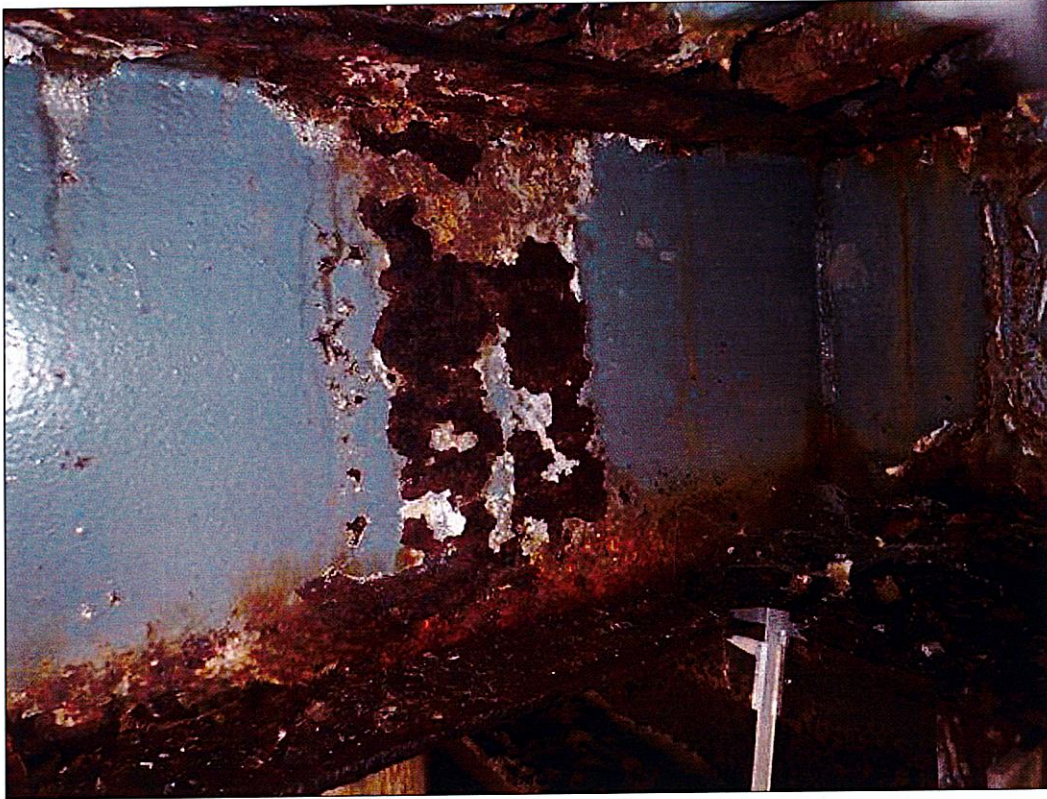
Span 1 Beam 3: 4 FEET OF RUST SCALE IN TOP AND BOTTOM FLANGES AND UP TO FULL HEIGHT IN THE WEB AT END BENT 1 WITH 1/4 INCHES REMAINING IN THE BOTTOM FLANGE, 1/4 INCHES REMAINING IN THE TOP FLANGE, AND 5/16 INCHES REMAINING IN THE WEB. (MUNICIPAL PAR)
