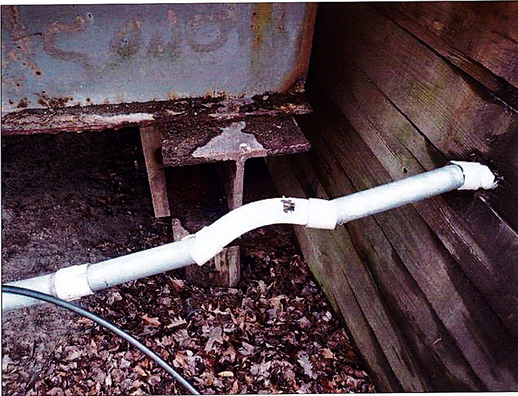
3 INCH DIAMETER METAL UTILITY IN THE NORTH END IS SAGGING AT MID SPAN AND HAS BROKEN CONNECTORS AT ENDS.
