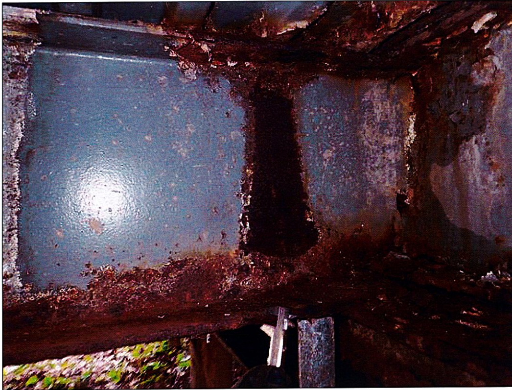
Span 1 Beam 7: 3.5 FEET OF RUST SCALE IN TOP AND BOTTOM FLANGES AT END BENT 1 WITH 5/16 INCHES REMAINING IN THE BOTTOM FLANGE AND NO MEASURABLE SECTION LOSS IN THE TOP FLANGE. (MUNICIPAL PAR)
