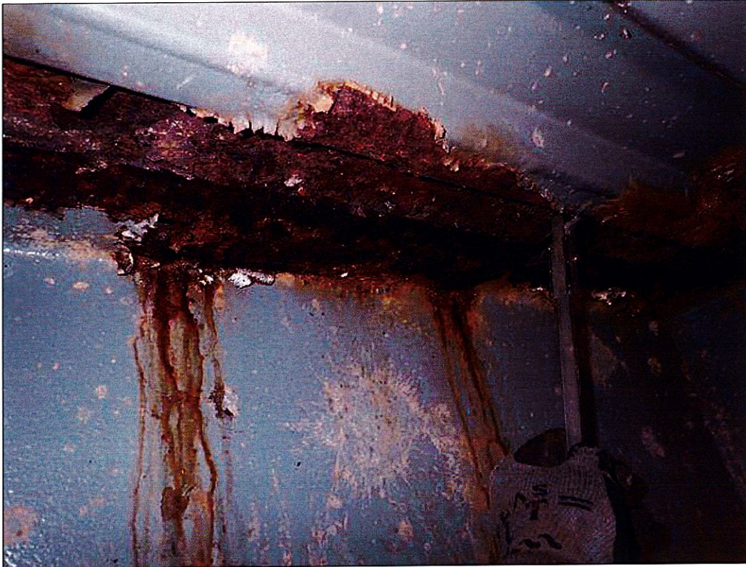
Span 1 Beam 7: RUST SCALE ON TOP FLANGE OF END DIAPHRAGM BETWEEN BEAMS 7 AND 8 AT END BENT 1 WITH 5/16 INCHES REMAINING. (MUNICIPAL PAR)
