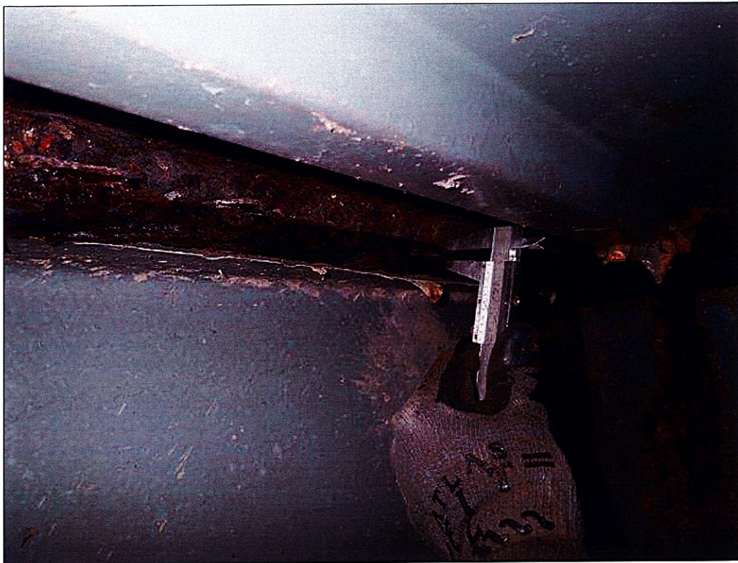
Span 1 Beam 8: RUST SCALE ON TOP FLANGE OF END DIAPHRAGM BETWEEN BEAMS 8 AND 9 AT END BENT 1 WITH 5/16 INCHES REMAINING. (MUNICIPAL PAR)
