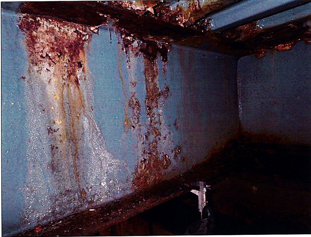
Span 1 Beam 2: 4 FEET OF RUST SCALE IN TOP AND BOTTOM FLANGES AND UP TO FULL HEIGHT IN THE WEB AT END BENT 1 WITH 1/4 INCHES REMAINING IN THE BOTTOM FLANGE, 3/16 INCHES REMAINING IN THE TOP FLANGE, AND 1/4 INCHES REMAINING IN THE WEB. (MUNICIPAL PAR)
