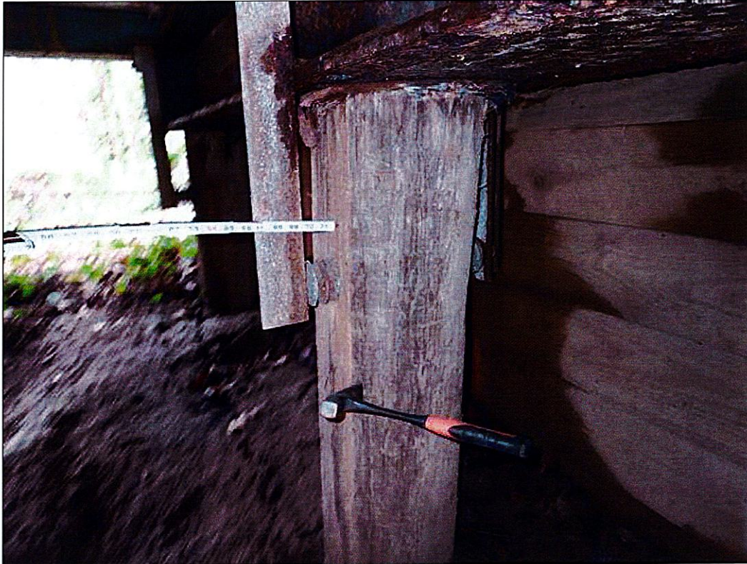
End Bent 1 Pile 5: EAST FACE HAS BEEN GROUND UP TO 3/4 INCHES TO SQUARE THE FACE TO THE CAP.
