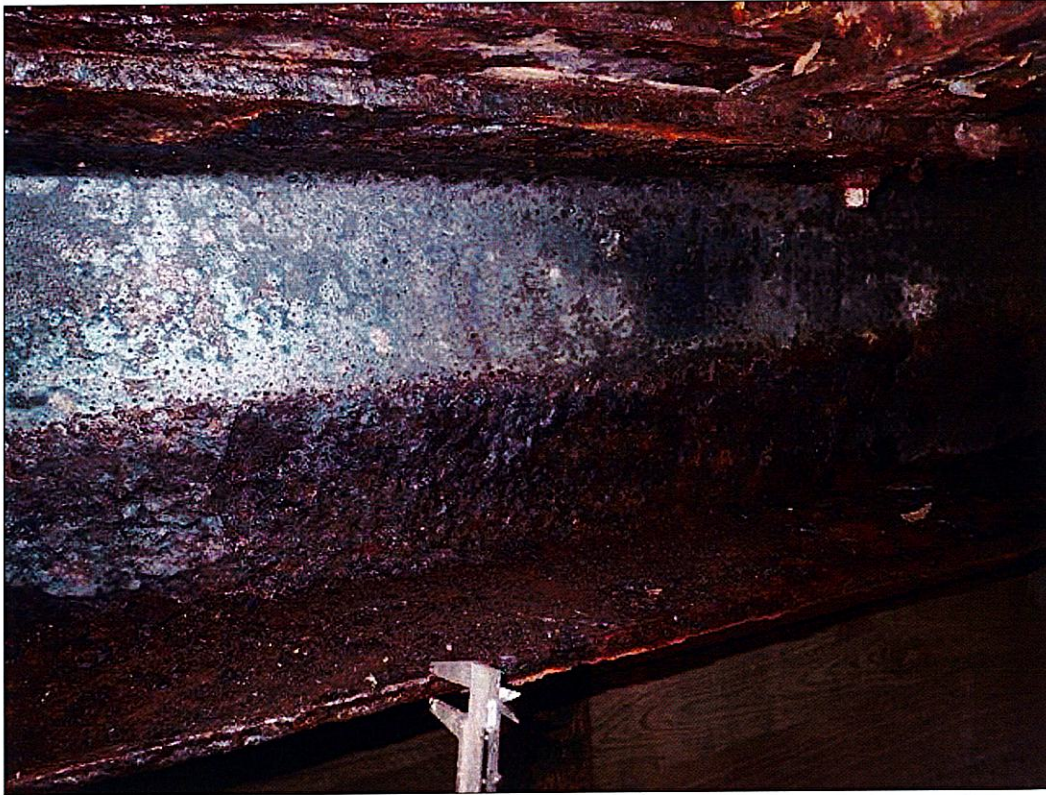
End Bent 2 Cap 1: CORROSION WITH SECTION LOSS IN THE TOP FLANGE, WEB, AND BOTTOM FLANGE BETWEEN PILES 1 AND 5. 5/8 INCHES THICKNESS REMAINS IN THE FULL WIDTH OF THE TOP AND BOTTOM FLANGES. 5/8 INCHES THICKNESS REMAINS IN THE FULL HEIGHT OF THE WEB. (MUNICIPAL PAR)
