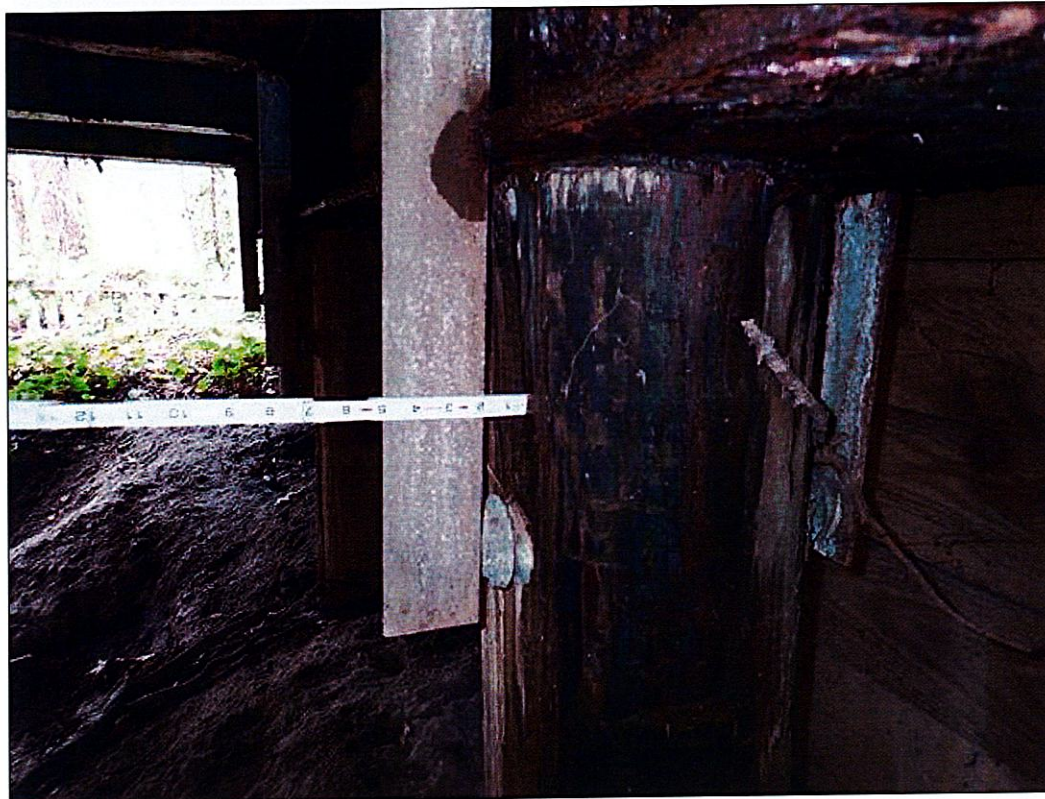
End Bent 1 Pile 4: CHECKS UP TO 3/4 INCHES.
