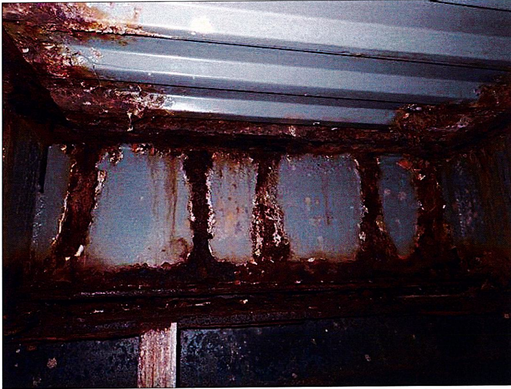
Span 1 Beam 4: RUST SCALE ON TOP AND BOTTOM FLANGES OF END DIAPHRAGM AT END BENT 2 WITH 5/16 INCHES REMAINING IN THE TOP FLANGE AND 3/16 INCHES REMAINING IN THE BOTTOM FLANGE. (MUNICIPAL PAR)
