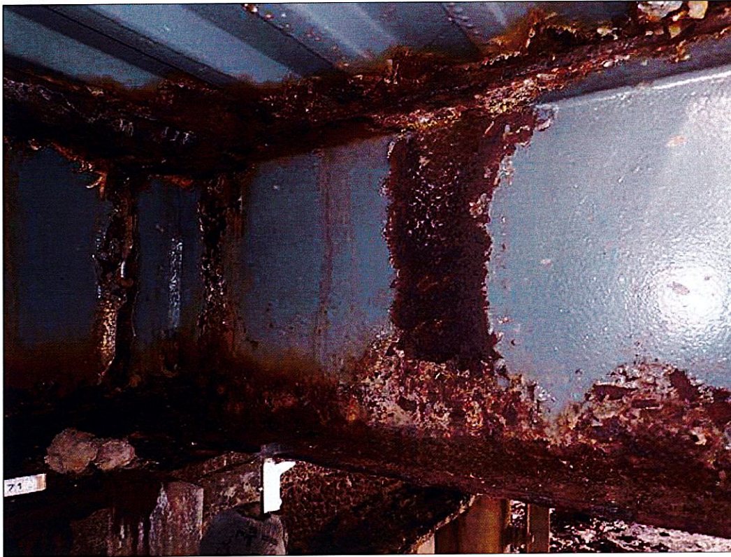
Span 1 Beam 4: 4.5 FEET OF RUST SCALE IN TOP AND BOTTOM FLANGES AND UP TO 4 INCHES IN THE WEB AT END BENT 1 WITH 5/16 INCHES REMAINING IN THE BOTTOM FLANGE, 3/8 INCHES REMAINING IN THE TOP FLANGE, AND NO MEASURABLE SECTION LOSS IN THE WEB. (MUNICIPAL PAR)
