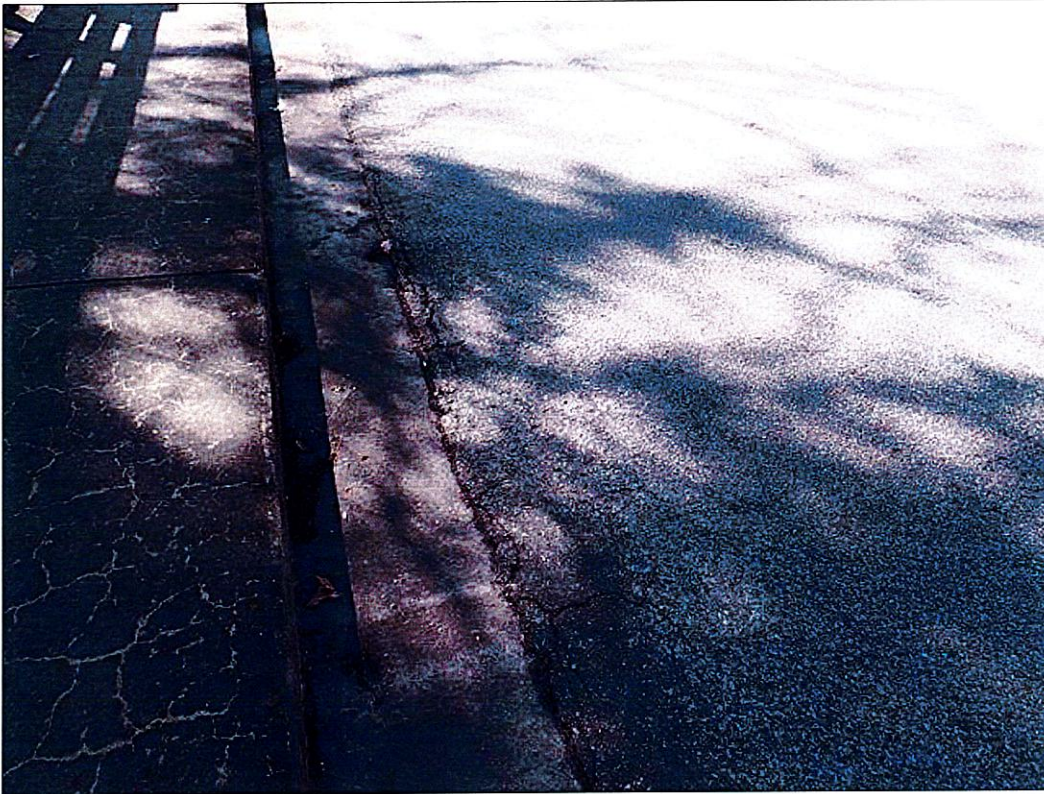
Span 1 Wearing Surface: 1/32 INCHES MAP CRACKING SCATTERED THROUGHOUT.
