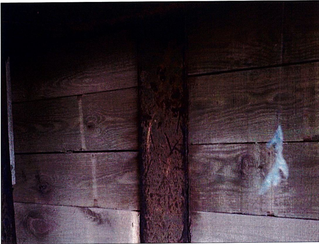
End Bent 1 Abutment: STEEL SOLDIER PILES IN THE ABUTMENT HAVE SURFACE CORROSION, NO SECTION LOSS.
