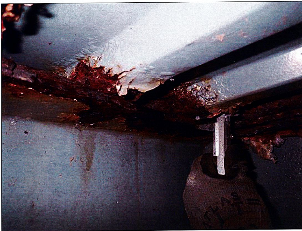
Span 1 Beam 8: 2 FEET OF RUST SCALE IN TOP FLANGE AT END BENT 2 WITH 5/16 INCHES REMAINING. (MUNICIPAL PAR)
