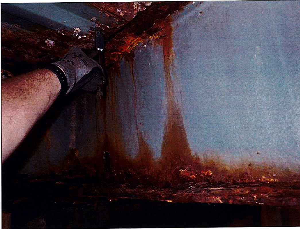
Span 1 Beam 3: 5 FEET OF RUST SCALE IN TOP AND BOTTOM FLANGES AND UP TO 5 INCHES IN THE WEB AT END BENT 2 WITH 3/8 INCHES REMAINING IN THE BOTTOM FLANGE, 3/16 INCHES REMAINING IN THE TOP FLANGE, AND NO MEASURABLE SECTION LOSS IN THE WEB. (MUNICIPAL PAR)
