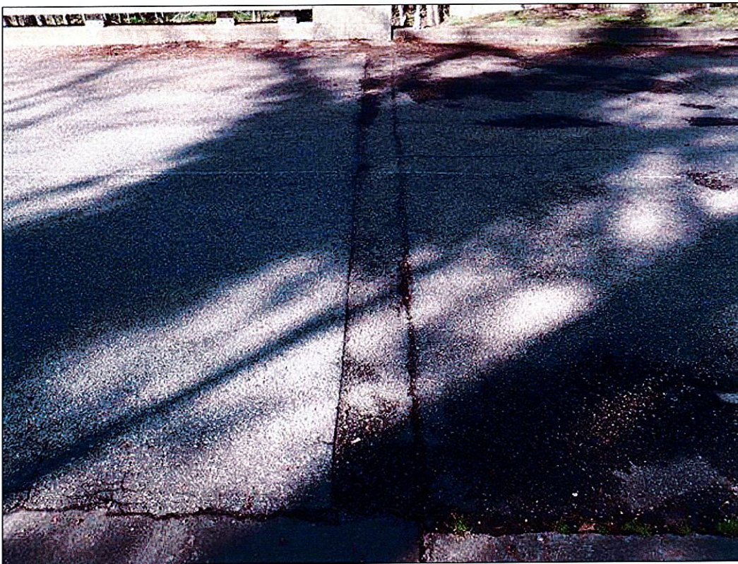
Span 2 Wearing Surface: TWO FULL WIDTH X 3/4 INCHES TRANSVERSE CRACKS ALONG END BENT 2 FILL FACE
