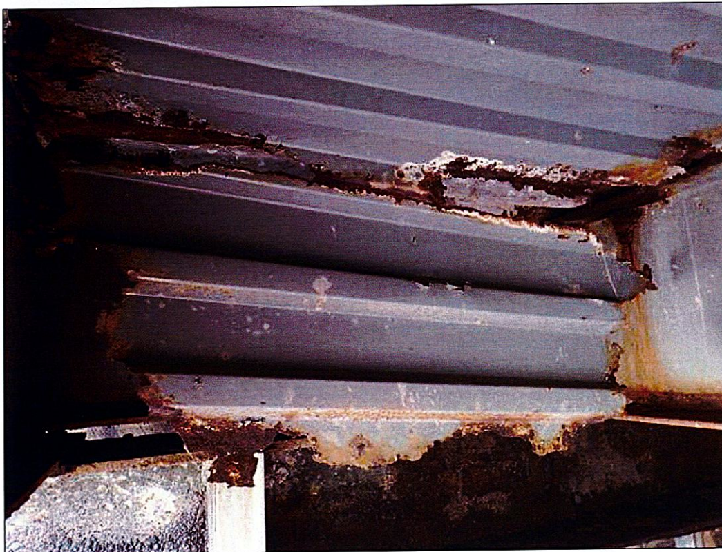
STAY-IN-PLACE FORM HAS SECTION HANGING 42" LONG X 16" WIDE IN BAY 2 AT END BENT 2
