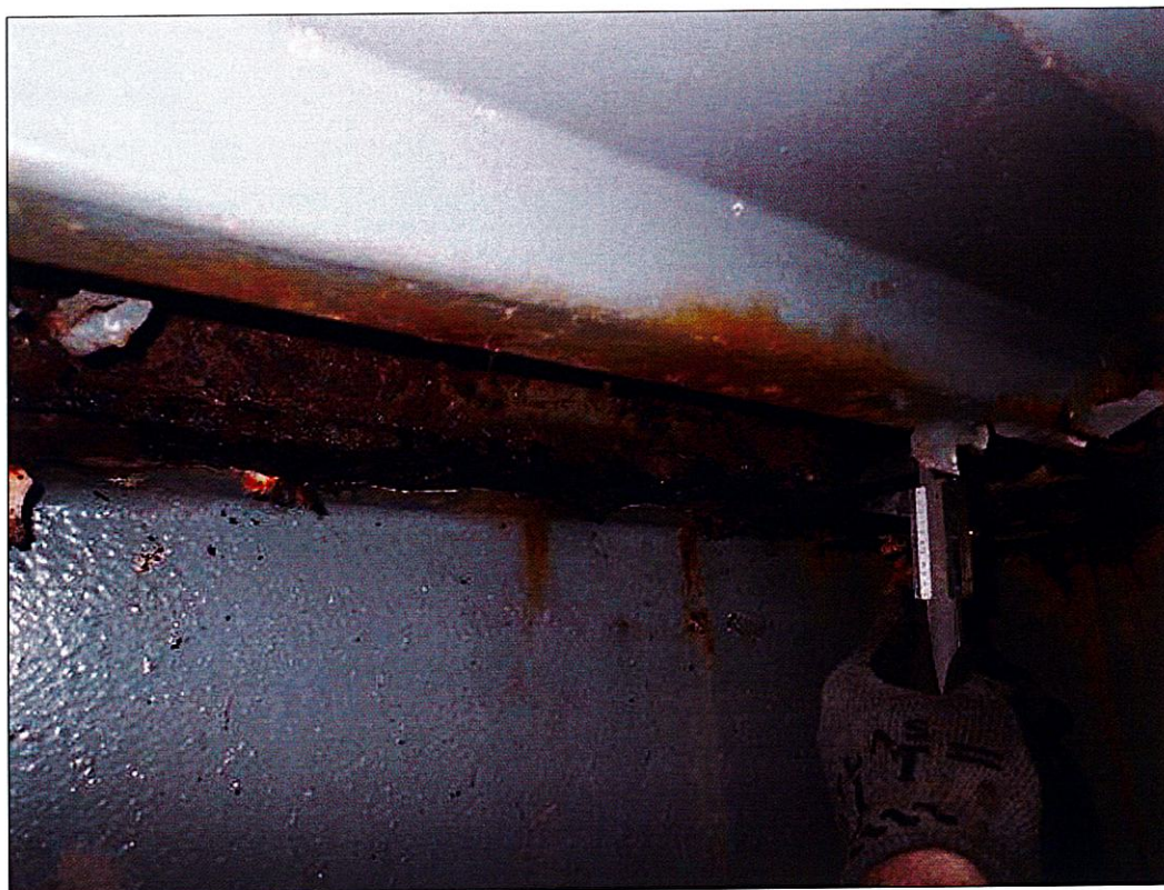
Span 1 Beam 1: RUST SCALE ON TOP FLANGE OF END DIAPHRAGM BETWEEN BEAMS 1 AND 2 AT END BENT 1 WITH 1/4 INCHES REMAINING. (MUNICIPAL PAR)
