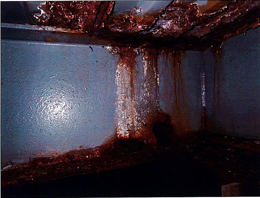
Span 1 Beam 7: 2.5 FEET OF RUST SCALE IN TOP AND BOTTOM FLANGES AT END BENT 2 WITH 5/16 INCHES REMAINING IN THE BOTTOM FLANGE AND 1/4 INCHES REMAINING IN THE TOP FLANGE. (MUNICIPAL PAR)
