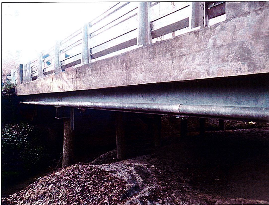
6 INCH DIAMETER UTILITY BELOW SOUTH OVERHANG
