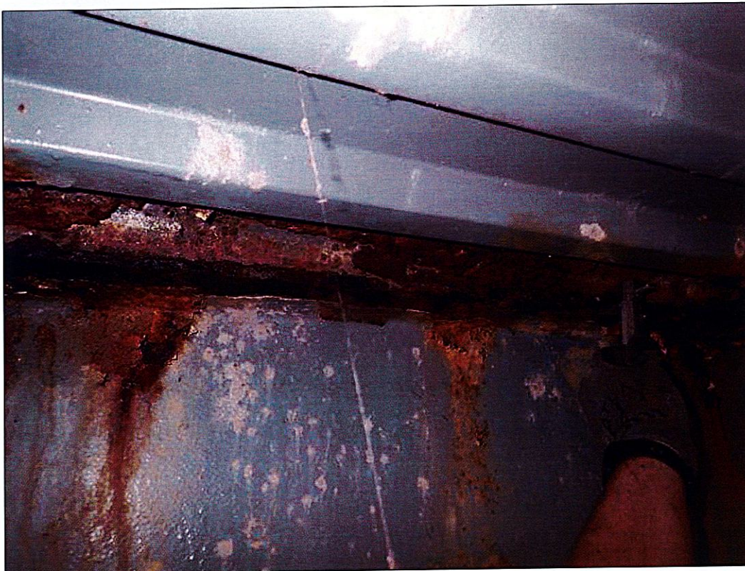
Span 1 Beam 2: RUST SCALE ON TOP FLANGE OF END DIAPHRAGM AT END BENT 2 WITH 5/16 INCHES REMAINING. (MUNICIPAL PAR)
