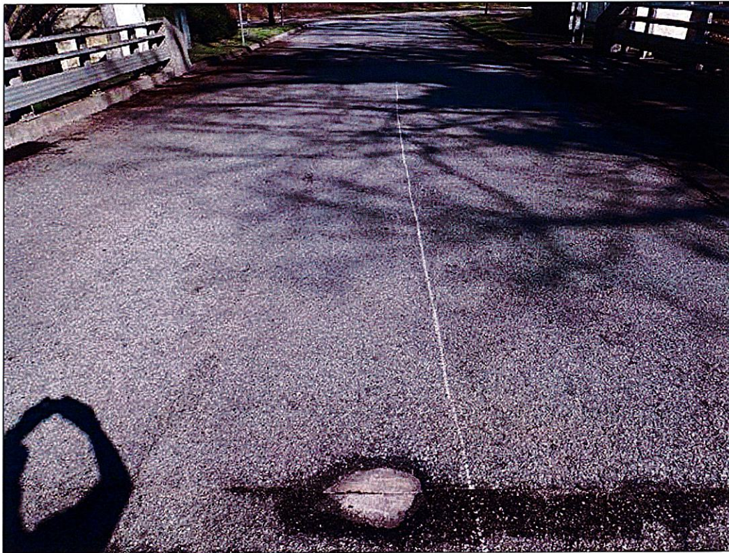
ASPHALT WEARING SURFACE, TYPICAL
