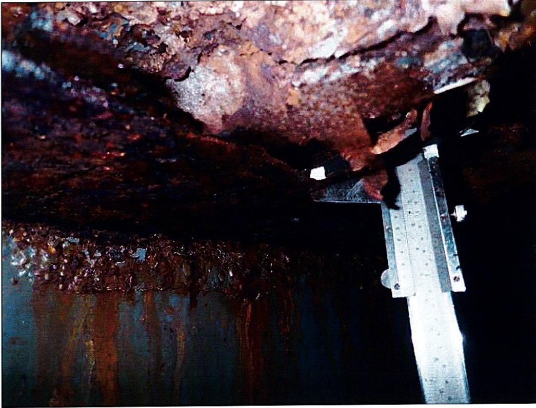
Span 1 Beam 5: 5.5 FEET OF RUST SCALE IN TOP AND BOTTOM FLANGES AND UP TO 5 INCHES IN THE WEB AT END BENT 2 WITH 1/4 INCHES REMAINING IN THE BOTTOM FLANGE, 1/8 INCHES REMAINING IN THE TOP FLANGE, AND 1/4 INCHES REMAINING IN THE WEB. (MUNICIPAL PAR)
