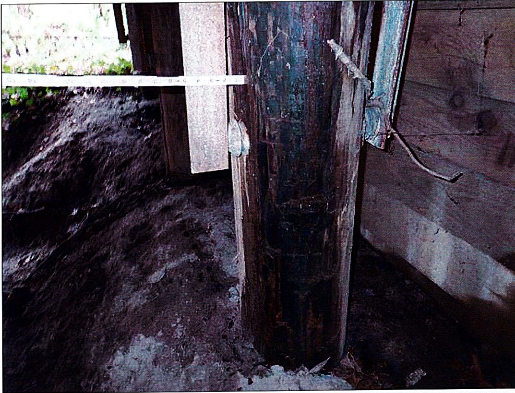
End Bent 1 Pile 4: EAST FACE HAS BEEN GROUND UP TO 1 INCHES TO SQUARE THE FACE TO THE CAP.
