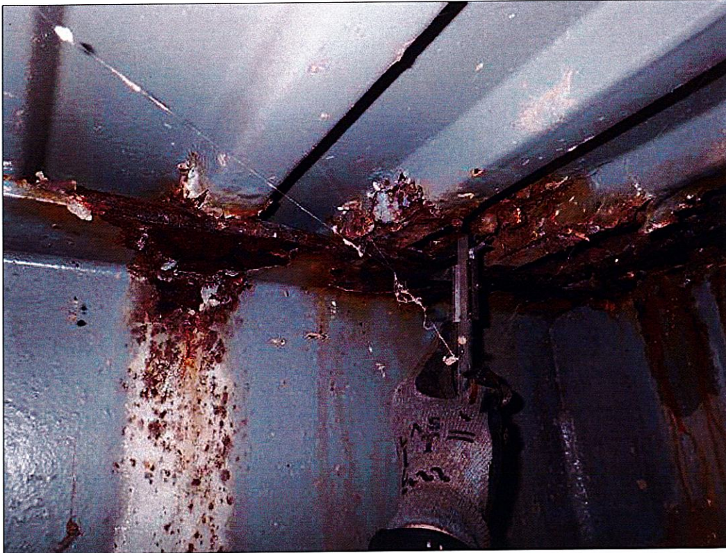
Span 1 Beam 8: 4 FEET OF RUST SCALE IN TOP AND BOTTOM FLANGES AND UP TO FULL HEIGHT IN THE WEB AT END BENT 1 WITH 5/16 INCHES REMAINING IN THE BOTTOM FLANGE, 1/4 INCHES REMAINING IN THE TOP FLANGE, AND NO MEASURABLE SECTION LOSS IN THE WEB. (MUNICIPAL PAR)
