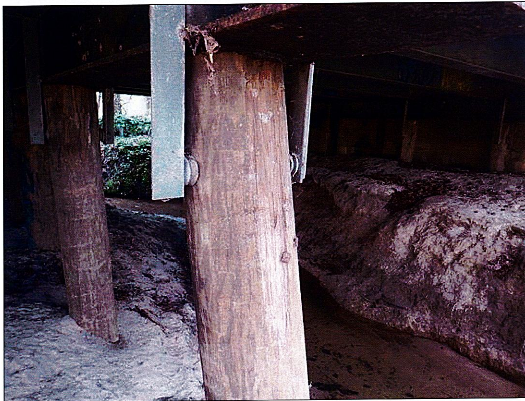
Bent 1 Pile 1: 5 INCHES WIDE X 26 INCHES HIGH X 1 INCHES DEEP SHAKE ON SOUTH FACE AT BOTTOM OF CAP. FULL HEIGHT ON NORTH FACE
