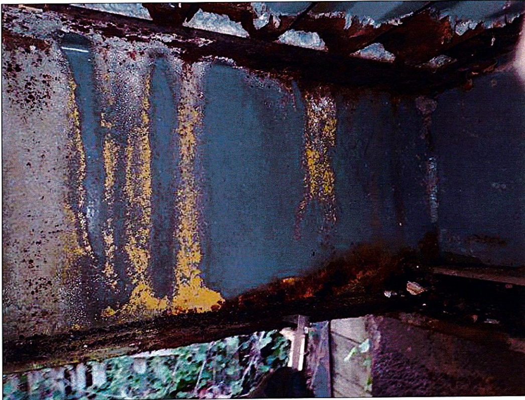
Span 1 Beam 9: 2.5 FEET OF RUST SCALE IN TOP AND BOTTOM FLANGES AT END BENT 1 WITH 1/4 INCHES REMAINING IN THE BOTTOM FLANGE AND NO MEASURABLE SECTION LOSS IN THE TOP FLANGE. (MUNICIPAL PAR)
