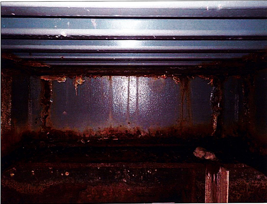
Span 1 Beam 4: LIGHT SCALING ON TOP AND BOTTOM FLANGES OF END DIAPHRAGM BETWEEN BEAMS 4 AND 5 AT END BENT 1.
