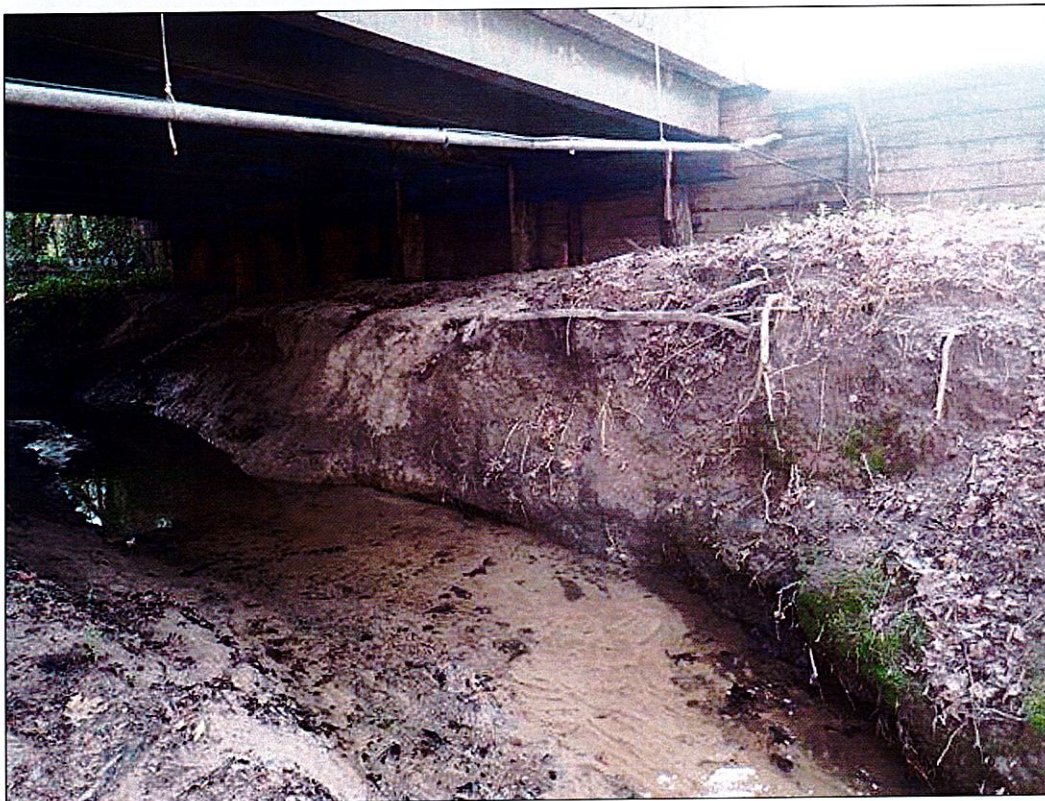
BANK EROSION UNDER SPAN 1. BANKS ARE VERTICAL UP TO 6 FEET TALL AND BEGINNING TO SLUMP FOR 50 FEET UPSTREAM AND DOWNSTREAM OF BRIDGE.
