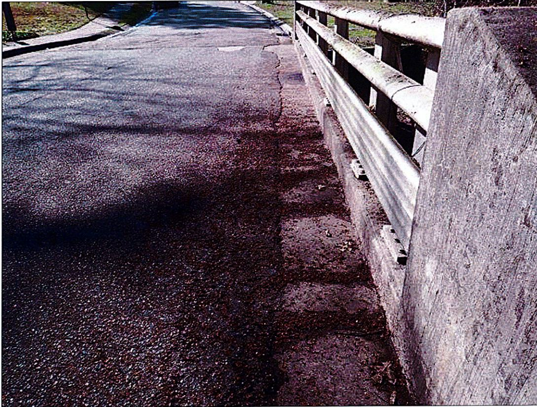
Span 2 Deck: EXPOSED SHOULDERS IN THE TOP OF THE DECK HAS SCATTERED TRANSVERSE HAIRLINE CRACKS UP TO 1.5 FEET LONG
