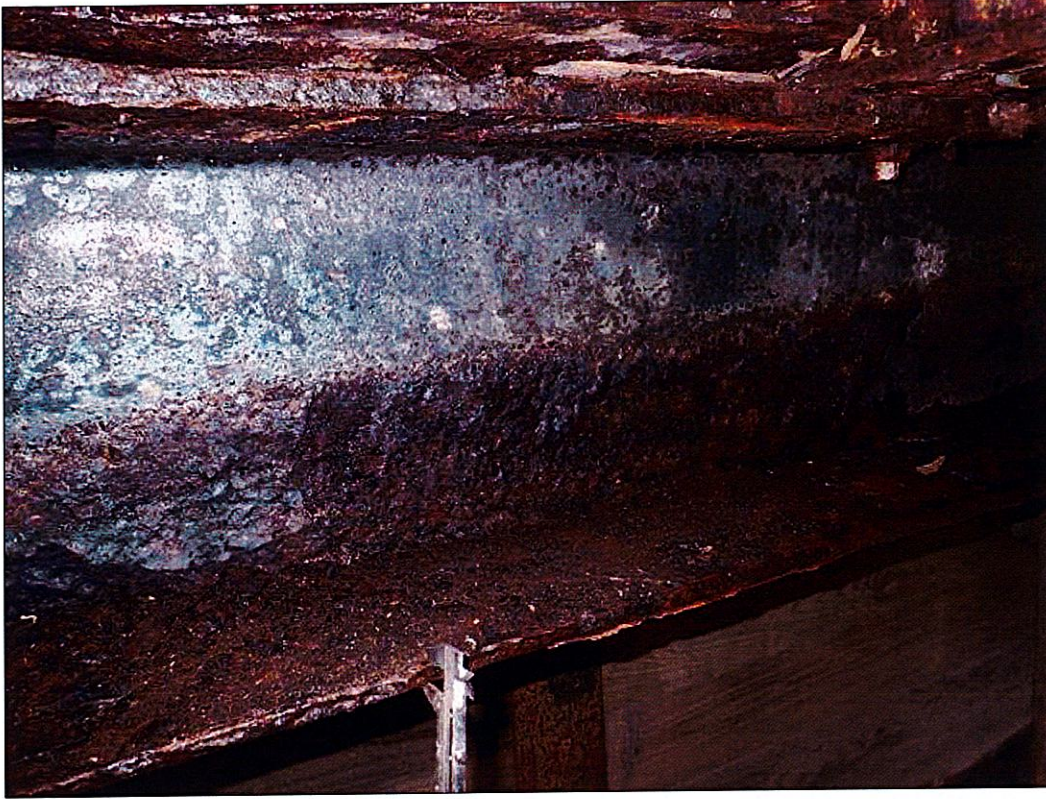
End Bent 1 Cap 1: CORROSION WITH SECTION LOSS IN THE TOP FLANGE, WEB, AND BOTTOM FLANGE BETWEEN PILES 1 AND 6. TOP AND BOTTOM FLANGES HAVE 1/2 INCHES THICKNESS REMAINING OVER THE FULL WIDTH. WEB HAS 5/8 INCHES THICKNESS REMAINING IN THE LOWER 6 INCHES. (MUNICIPAL PAR)
