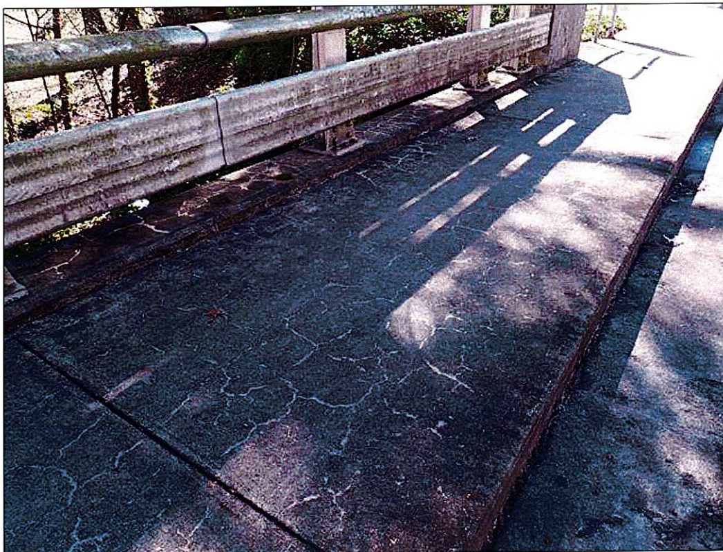
Span 1 Deck: TOP OF CURB AND SIDEWALK HAVE HAIRLINE MAP CRACKING WITH EFFLORESCENCE FOR THE FULL LENGTH.
