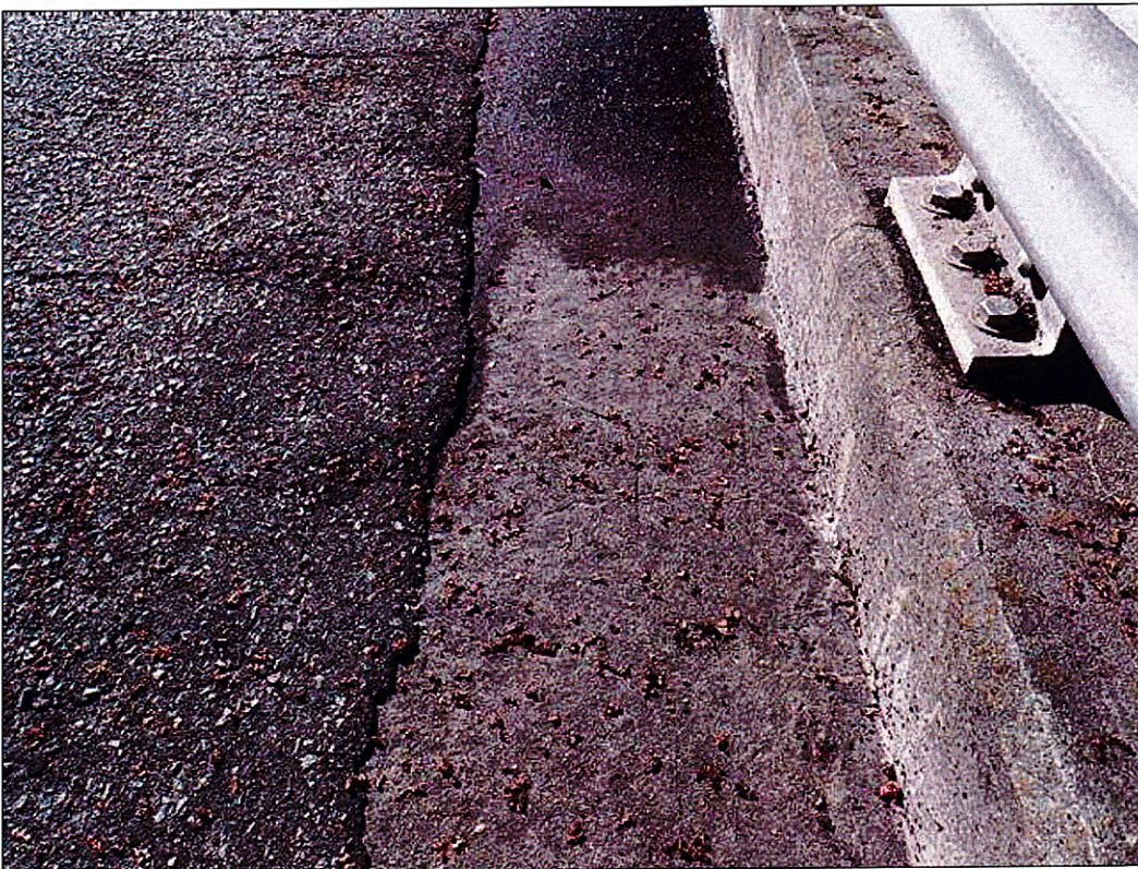
Span 1 Deck: EXPOSED LEFT SHOULDERS IN THE TOP OF THE DECK HAS SCATTERED TRANSVERSE HAIRLINE CRACKS UP TO 1.5 FT LONG
