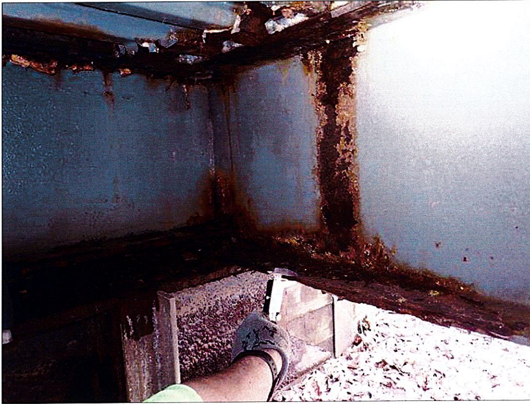
Span 1 Beam 1: 4 FEET OF RUST SCALE IN TOP AND BOTTOM FLANGES WITH UP TO FULL HEIGHT LIGHT SCALING IN THE WEB AT END BENT 1 WITH 1/4 INCHES REMAINING IN THE BOTTOM FLANGE, 3/8 INCHES REMAINING IN THE TOP FLANGE, AND NO MEASURABLE SECTION LOSS IN THE WEB. (MUNICIPAL PAR)
