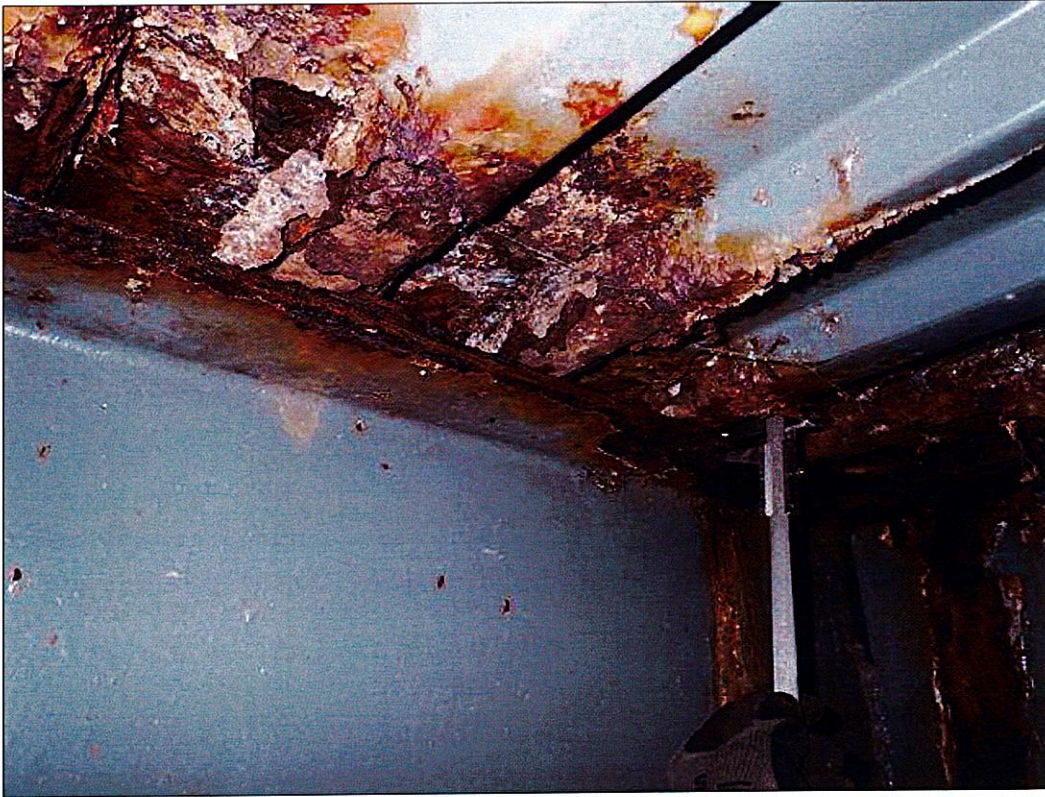
Span 1 Beam 4: 6 FEET OF RUST SCALE IN TOP AND BOTTOM FLANGES AND UP TO 6 INCHES IN THE WEB AT END BENT 2 WITH 1/4 INCHES REMAINING IN THE BOTTOM FLANGE, 1/4 INCHES REMAINING IN THE TOP FLANGE, AND 1/4 INCHES REMAINING IN THE WEB. (MUNICIPAL PAR)
