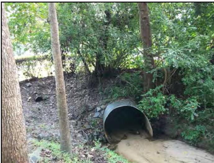
Picture 4-3. Upstream Invert – Oxford Road Closed System (Bells Branch)
