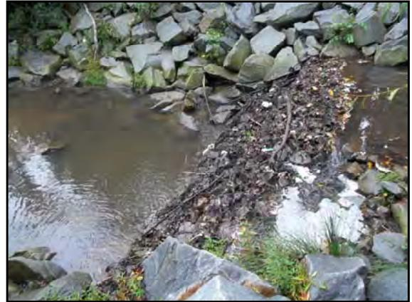
Picture 5-3. Existing rock drop structure
