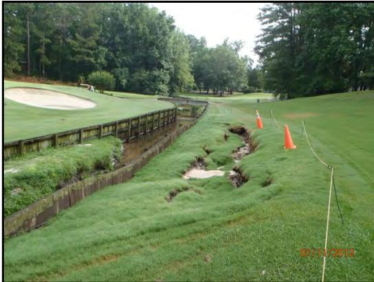
**Picture 5-6.** Right bank area sinking behind retaining wall along the Brook Valley Golf Course Project
