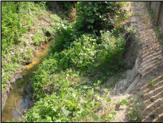
**Picture 5-2.** Severe bank erosion along landscaping fence
