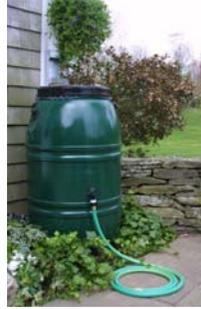
Rain barrels or cisterns can store rain water for irrigation or wash water for vehicles.
