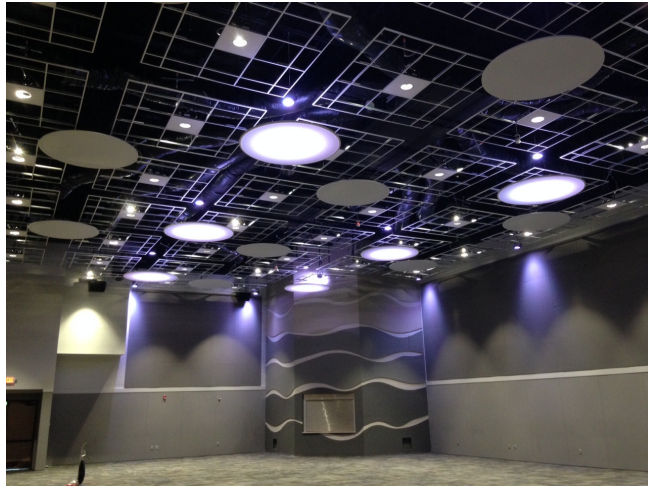
Figure 1 - Exhibit Hall Cloud Ceiling being installed
