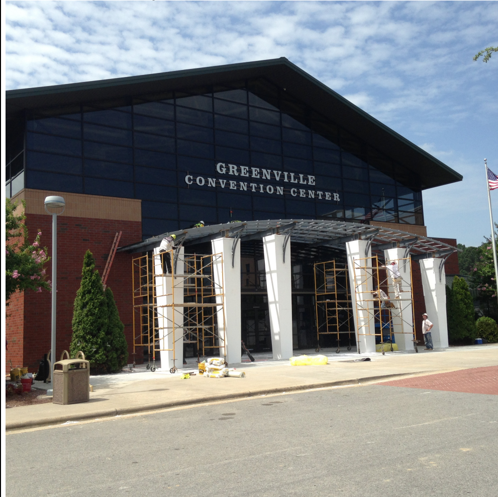
Figure 1 – New Front Entrance Canopy Installation
