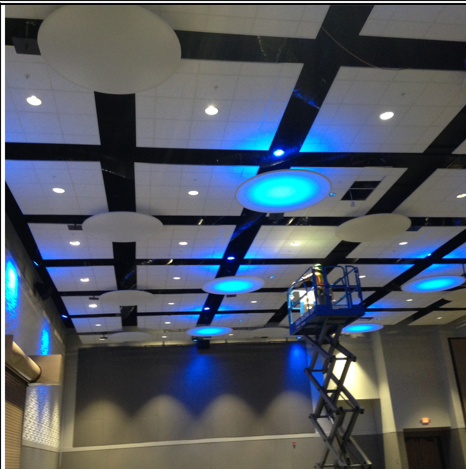
Figure 2 - Exhibit Hall Cloud Ceiling being installed
